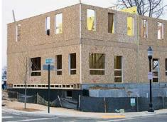
SIP walls and open-webbed floor trusses expedited on-site construction. Floor trusses, however, increased potential leakage areas at the rim joist, and were carefully air sealed with spray foam.
