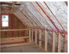
Nexus EnergyHomes used spray foam insulation to seal and insulate the attic as well as elastomeric sealant at key framing junctures to keep HVAC in conditioned space, add living space affordably, and tighten the building.
