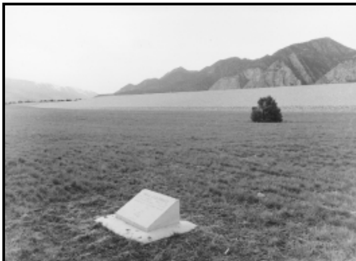
Estes Gulch Disposal Cell Marker identifying the site of buried uranium mill tailings at Estes Gulch, near Rifle, Colorado. In addition to a scale map of the site, the inscription reads: "Rifle, Colorado. Date of Closure April 26, 1996. Dry tons of tailings 4,967,451. Radioactivity 2,738 Curies RA-226." Estes Gulch Disposal Cell, Rifle, Colorado, June 1998.
