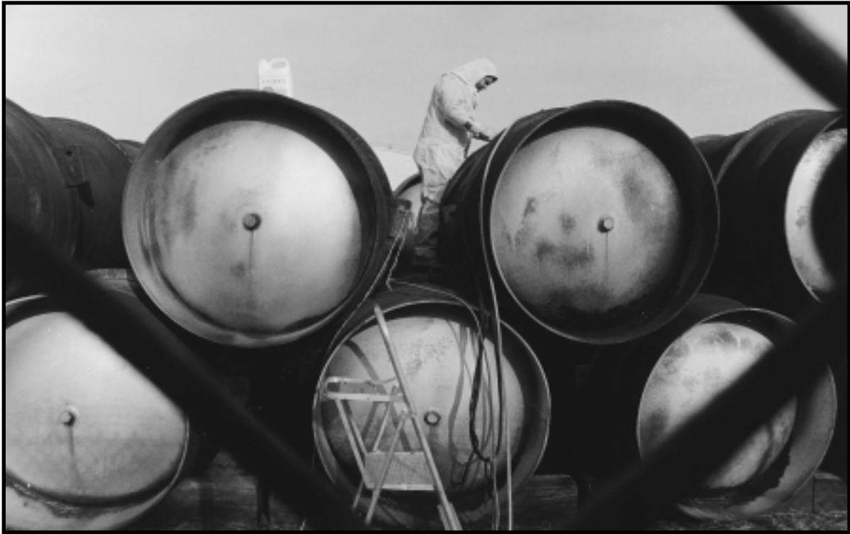
Maintenance of Uranium Hexafluoride Cylinders. A worker at the Oak Ridge Reservation uses ultrasound to evaluate the effects of corrosion on a steel cylinder containing depleted uranium hexafluoride — the material left over from the uranium enrichment process. DOE owns over 46,000 cylinders of this material weighing 10 to 14 tons each. By mass, depleted uranium makes up over 70 percent of the Department's Materials in Inventory. After decades of storing this material, the Department is now undertaking a conversion project to stabilize the uranium hexafluoride for final disposition. K-1066-K Cylinder yard, K-25 Site, Oak Ridge, Tennessee January 1994.
