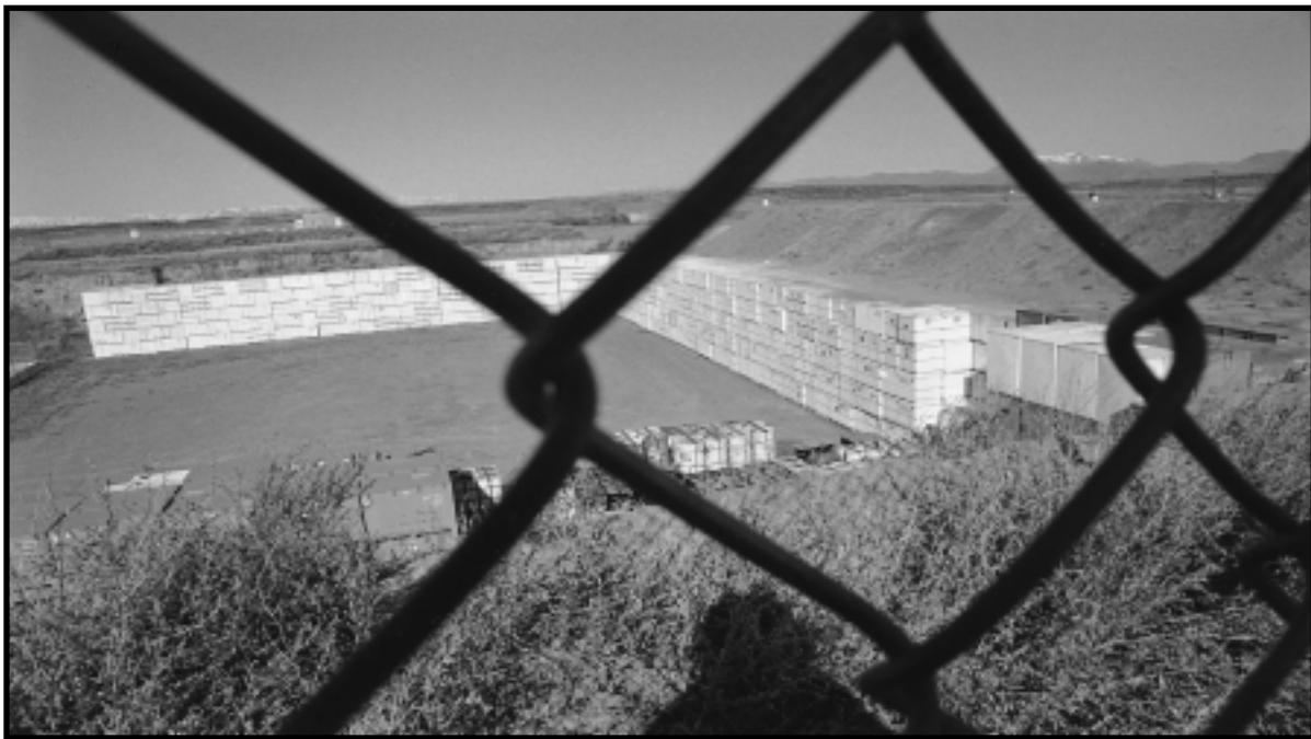
Low-Level Waste Burial. The Idaho National Engineering and Environmental Laboratory disposes of low-level waste in this pit at the Radioactive Waste Management Complex Subsurface Disposal Area. The laboratory has 4,700 cubic meters of low-level waste in inventory and is projected to generate an additional 115,000 cubic meters in the next 35 years. New waste will come from facility decommissioning and dismantlement, treating and characterizing other waste streams, and ongoing processes. Radioactive Waste Management Complex, Idaho National Engineering and Environmental Laboratory, Idaho, March 1994.
