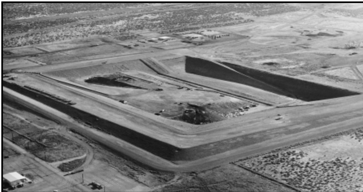
The Environmental Restoration Disposal Facility. This engineered unit receives waste generated by the Hanford site cleanup. Its bottom is lined with multi-layer high-density polyethylene. When full, the facility will be covered with a RCRA-compliant multi-layer cap, a vegetative cover, and a five-meter intrusion barrier made of basalt, concrete, boulders, silty soil, and plastic. Between its opening in 1996 and 1999, the site has taken in more than 1.6 million tons of contaminated soils and material. It is expected to close in 2046. Access to waste disposal areas and buffer zones will be restricted for as long as necessary to protect human health and the environment. Environmental Restoration Disposal Facility, Hanford Site, Washington, July 1998.
