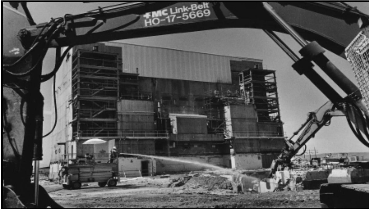
Preparation for Entombment. Before the Hanford “C” reactor core is entombed within its shielding walls, related structures are first decontaminated and dismantled. Contaminated soils and materials from the area have been disposed of in the Environmental Restoration Disposal Facility (below). Once entombed, the reactor core will require monitoring and maintenance for up to 75 years until a decision is made on its final disposition. C Reactor, Hanford Site, Washington, July 1998.
