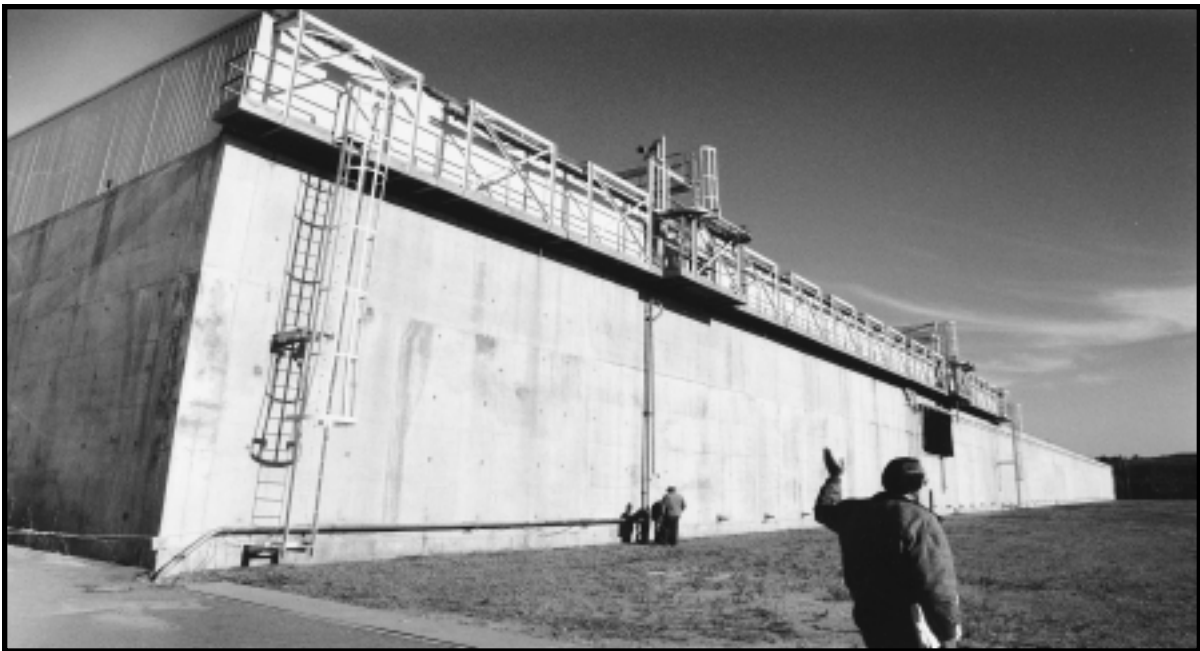
Low-Level Waste Disposal Vault. This vault for low-level waste is located at the Savannah River Site. It is a reinforced concrete structure 25 feet tall, 600 feet long, and 200 feet wide. It houses 12 concrete cells that will be filled with solid grout (“saltstone”) made by mixing a low-level waste solution with cement, fly ash, and slag. Radionuclides in the grout will include technetium-99, strontium-90, and cesium-137. Once all 12 cells are filled, the vault will be covered with earth and capped with clay. Active maintenance and monitoring will be required, along with passive institutional controls to prevent intrusion. Z-Area Vault, Savannah River Site, South Carolina, January 1994.
