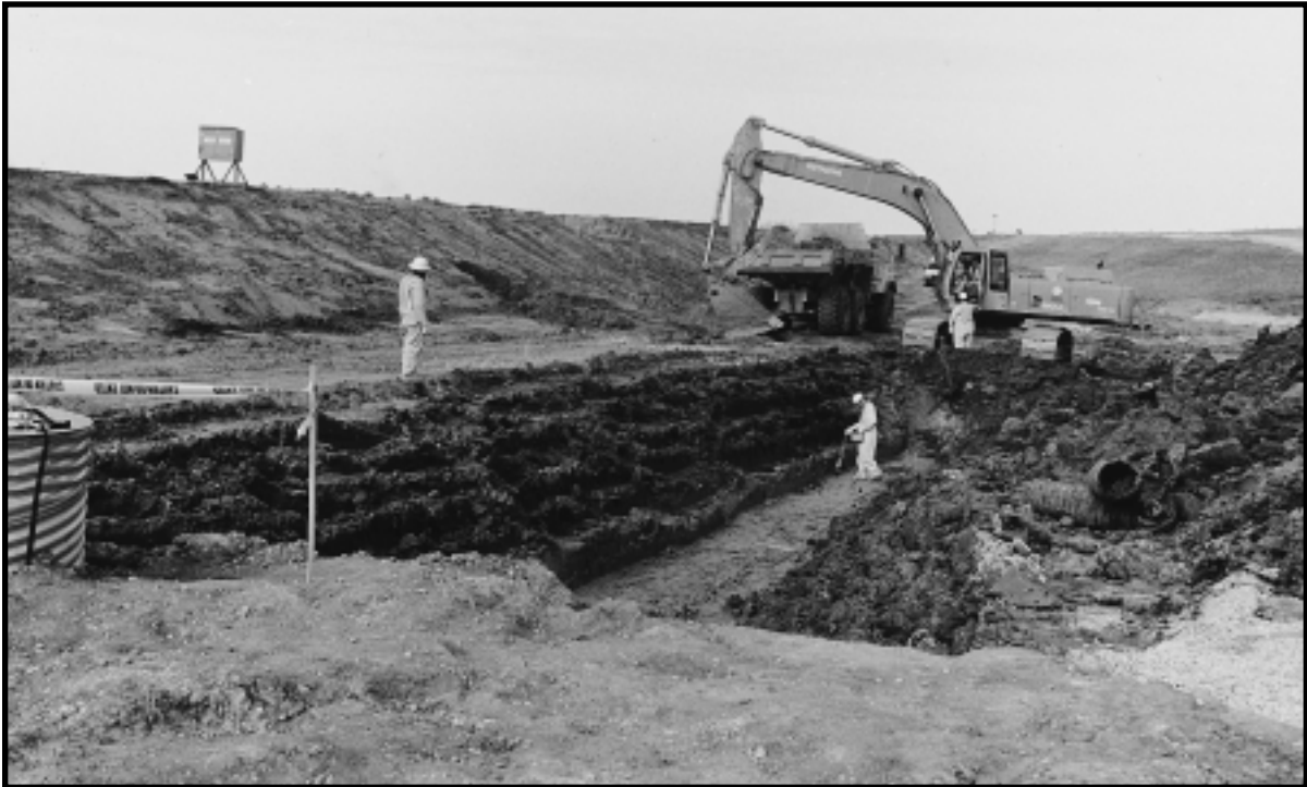
During: Weldon Spring Site Remedial Action Project. Remediation began at Weldon Spring in 1985 and involved dismantling the chemical plant buildings, excavating contaminated soils, and disposing of radioactive and chemically- contaminated soil and debris. Weldon Spring Site Remedial Action Project, near St. Louis, Missouri, March 1996.
