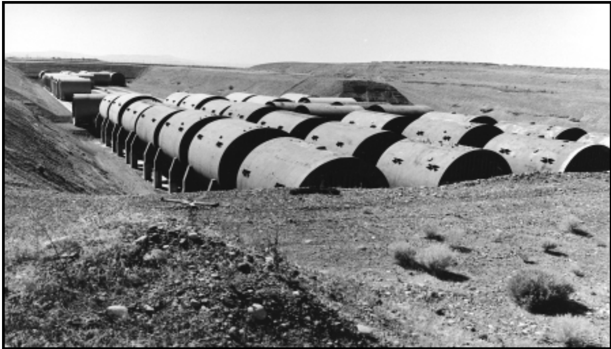
Submarine Hull Disposal Trench. When a nuclear-powered submarine is decommissioned, the spent nuclear fuel is removed from the submarine's reactors and the section of the submarine containing the reactor is disposed of in a trench. The radioactively-contaminated hull sections with the defueled reactors inside are transported by barge to the Hanford Site, where they are placed in a large trench for burial. The disposal trench will require long-term monitoring and maintenance to ensure that hazardous materials remain inside the hulls. Trench 94, Hanford Site, Washington, July 1998.
