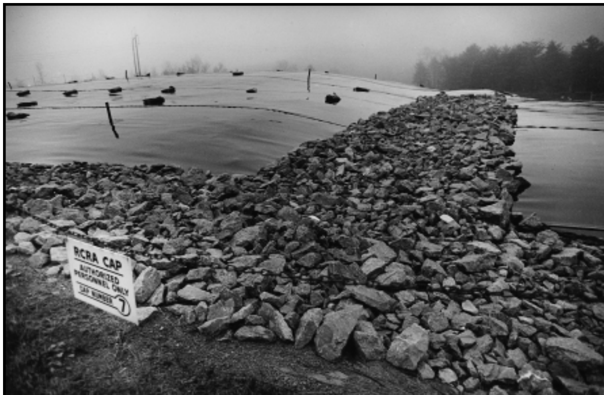
Landfill with RCRA Cap. Ten acres of black, high-density polyethylene cover a mixed waste landfill at the Oak Ridge Reservation. The cap is designed to prevent gases from escaping, reduce erosion, and keep rainwater from leaching contaminants into groundwater. Installed in 1989, the cap is designed to last from 15 to 20 years. Maintenance and monitoring will be required at least until 2019. Solid Waste Storage Area 6, Oak Ridge Reservation, Tennessee, January 1994.
