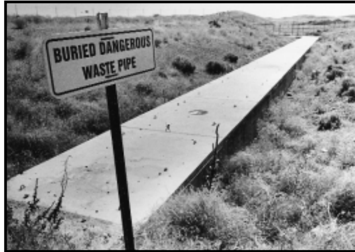
Buried Waste Pipe Sign indicating location of buried waste pipe. N Reactor Area, Hanford Site, Washington, July 1998.
