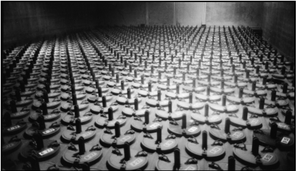
Irradiated Nuclear Fuel in Dry Storage. Spent nuclear fuel is a highly radioactive material that has not been reprocessed to remove the constituent elements. This waste must be stored in facilities that shield and cool the material. DOE plans to remove all spent nuclear fuel from the site by 2035 and dispose of it in the proposed geologic repository. Building 603, Idaho Nuclear Technology and Engineering Center, formerly the Idaho Chemical Processing Plant, Idaho National Engineering and Environmental Laboratory, Idaho, March 1994.
