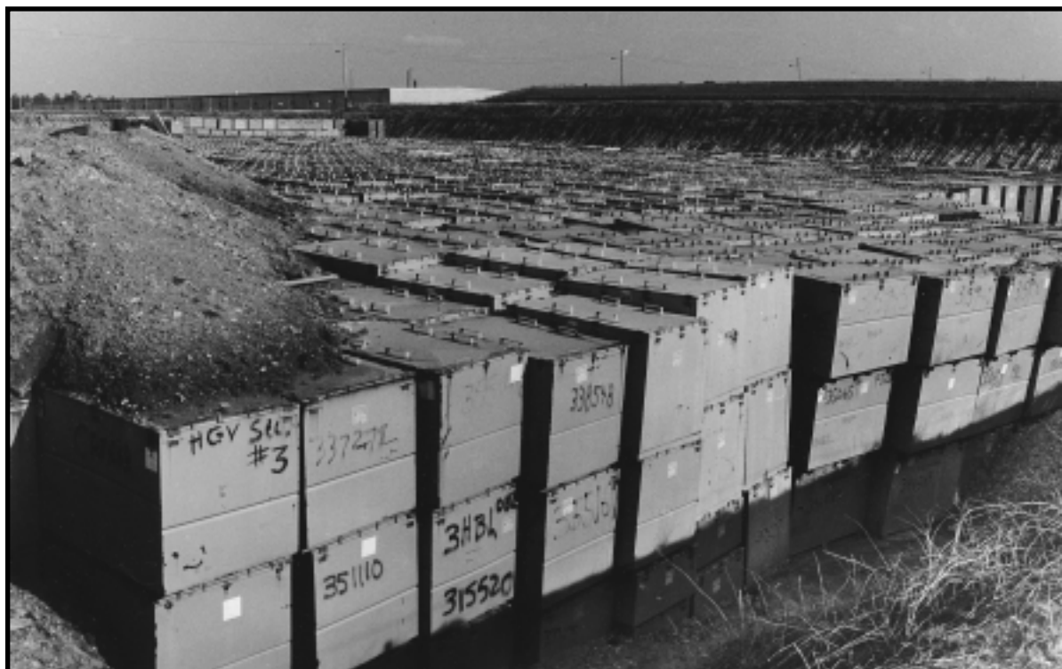
Low-Level Waste Disposal Site. This engineered trench at the Savannah River Site contains approximately 30,000 stacked carbon-steel boxes of waste with each box measuring 4 by 4 by 6 feet. In 1996 the trench was backfilled with dirt to form a mound, which was seeded with grasses and sloped to reduce runoff. Long-term monitoring and maintenance will be needed to ensure the integrity of this waste containment system. Engineered Low-Level Trench 4, Savannah River Site, South Carolina, January 1994.
