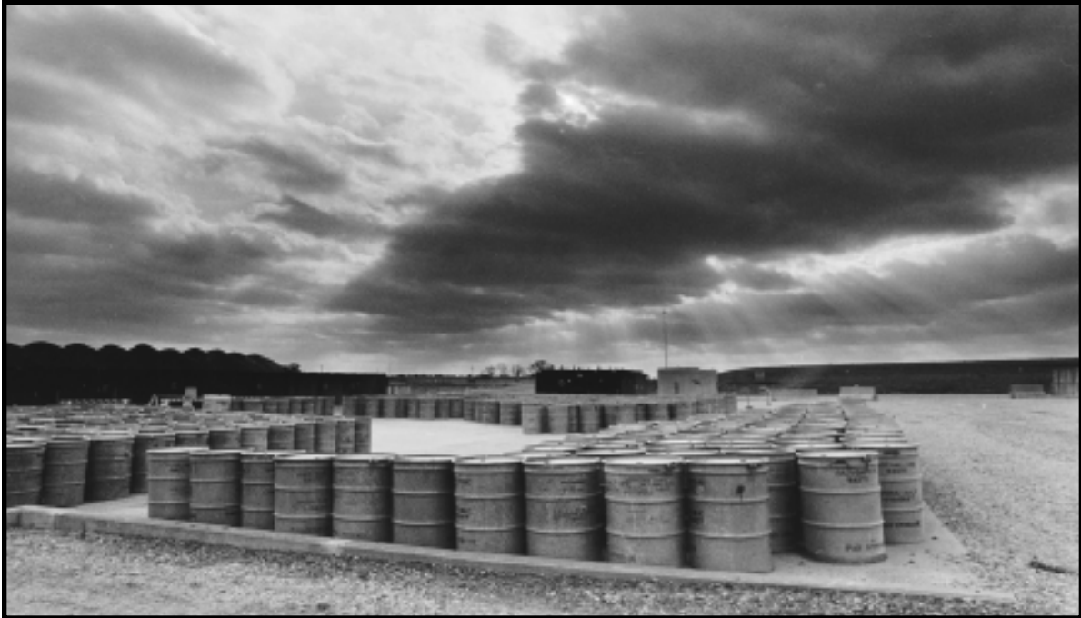
Transuranic Waste Storage Pads. Drums containing transuranic waste sit on a concrete pad in temporary storage. This waste is contaminated with uranium-233 and plutonium. In 1999, the Department began disposing of transuranic waste in the Waste Isolation Pilot Plant near Carlsbad, New Mexico. Transuranic Waste Storage Pads, E Area Burial Grounds, Savannah River Site, South Carolina, January 1994.
