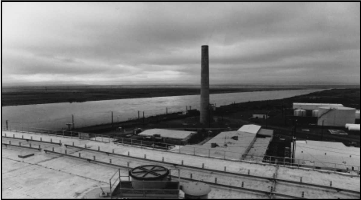
N Reactor along the Columbia River. Originally, the river provided cooling water for the reactor. Spent nuclear fuel has been stored in the “wet storage” (water filled) basins in this complex of buildings supporting the reactor, which ceased operations in 1987. Because of corrosion of the cladding of the spent fuel rods, approximately 15 million gallons of water contaminated with strontium-90 has been released into the groundwater. DOE has installed a groundwater pump-and-treat system to control the movement of the contaminated groundwater. Institutional controls will remain in place at the site indefinitely to restrict groundwater use, and the semi-annual monitoring will continue for at least 30 years after closure of the last facilities. N Reactor; Hanford Site, Washington, July 1994.
