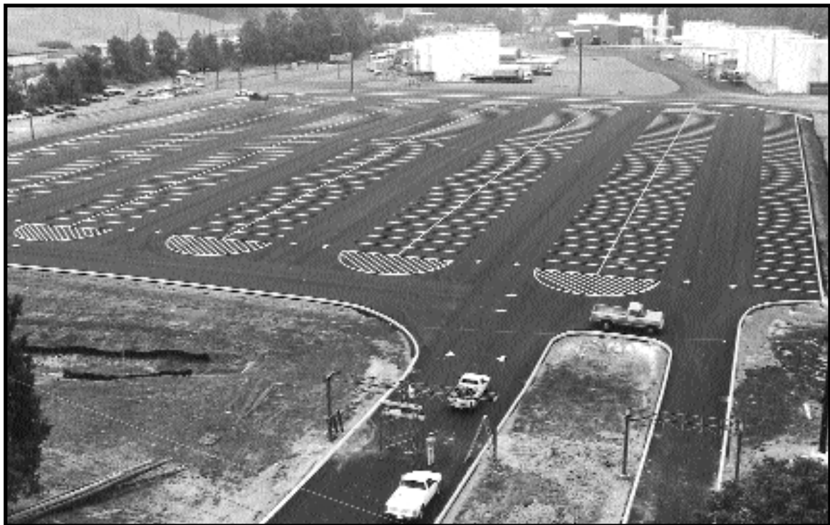
After. From 1985 until 1990, liquids in the above four waste ponds were treated to remove contaminants, the ponds were then drained and capped with asphalt, and the capped area used as a parking lot. The asphalt cap will require long-term monitoring and maintenance to ensure its integrity and prevent migration of the residual contamination beneath it. Oak Ridge Reservation, Tennessee. Photo circa 1990. Source: U.S. Department of Energy.
