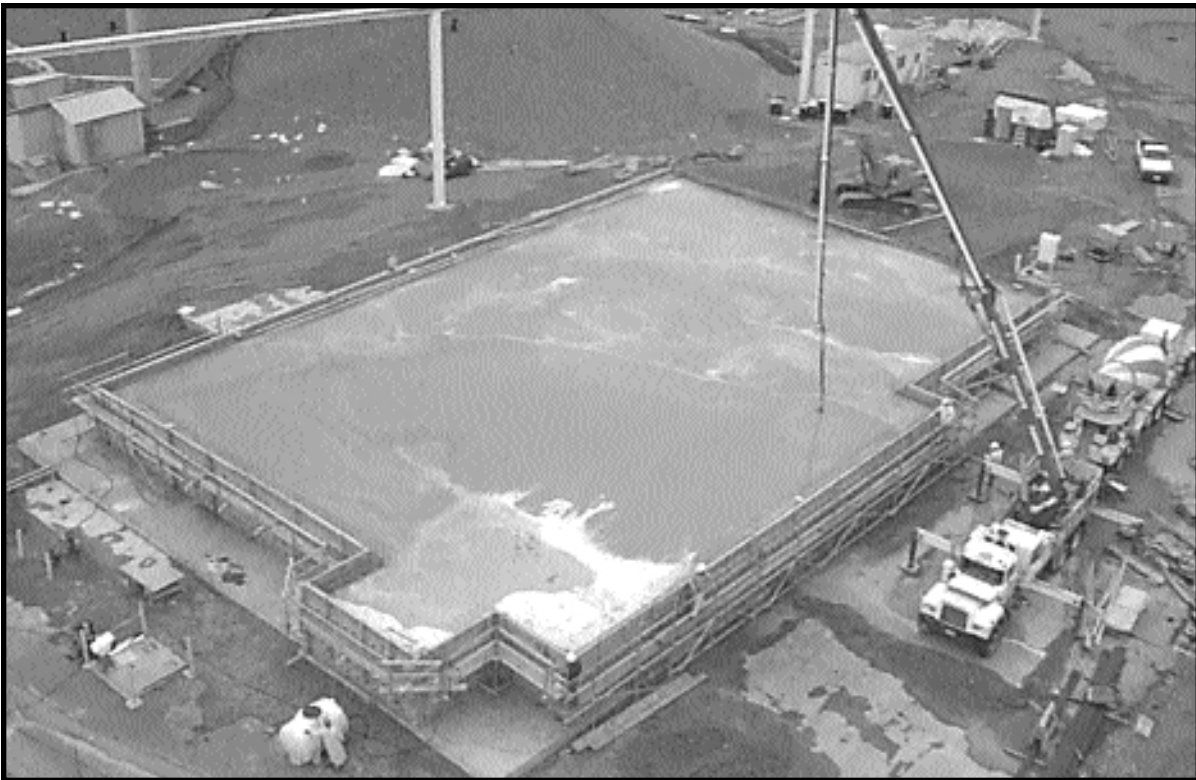
After: Waste Calcining Facility. After the calcining plant's superstructure and contaminated equipment had been demolished, the remaining rubble pile was filled with grout to stabilize any residual contamination. Idaho National Engineering and Environmental Laboratory, Idaho, May 1999. Source: U.S. Department of Energy - Idaho Operations.
