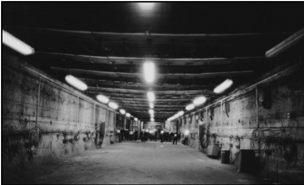
Underground Transuranic Waste Disposal Room. This room, excavated in 1986, is the first of 56 chambers to be excavated at the Waste Isolation Pilot Plant. It is 300 feet long, 33 feet wide, and 13 feet tall and can hold six thousand 55-gallon drums of transuranic waste. It lies 2,150 feet below the surface of the earth in an ancient stable salt formation. Room 1 of Panel 1, Waste Isolation Pilot Plant, New Mexico, February 1994.
