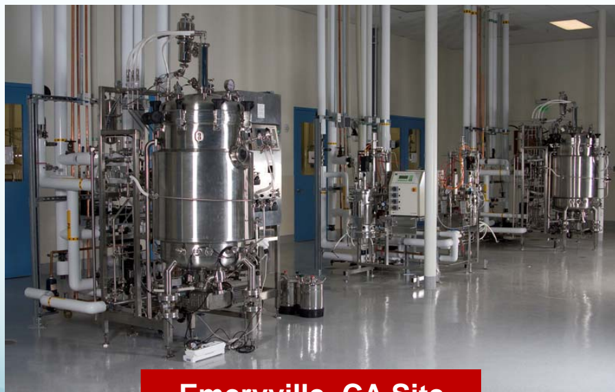
Emeryville, CA Site
