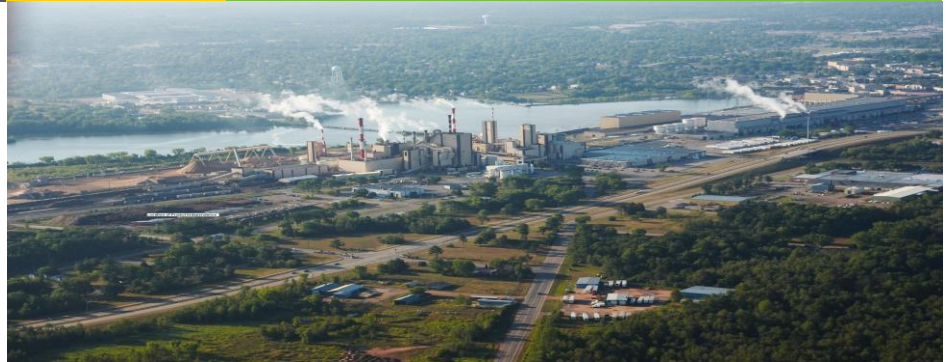
The integrated biorefinery in Wisconsin Rapids, Wisconsin, operated by NewPage.
