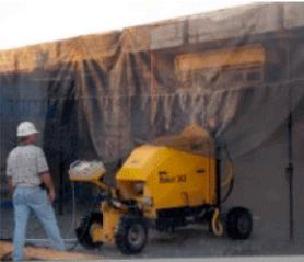
Figure 1. Conjet Robot 363 during ceiling hydrodemolition.
