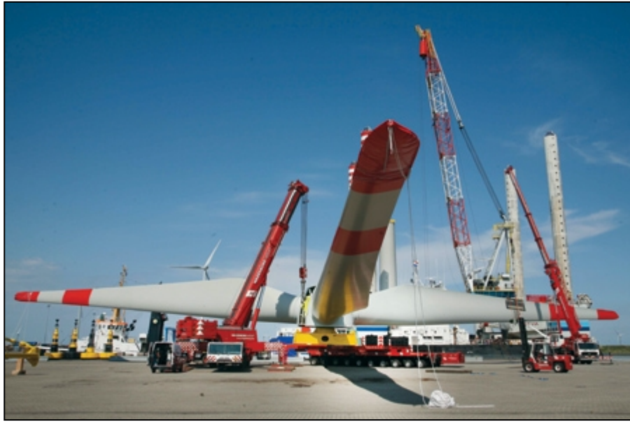
Figure 5-13: Full Rotor Assembly in Port
