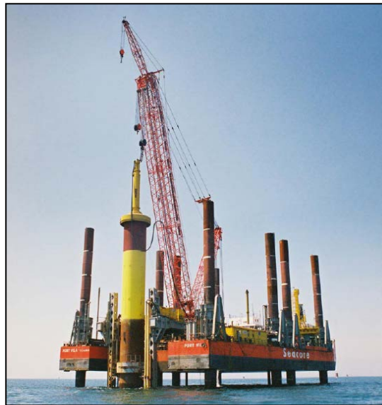
Figure 3-6: Steel Monopile being driven by a Menck Hydrohammer – Jack-up Excilbur
