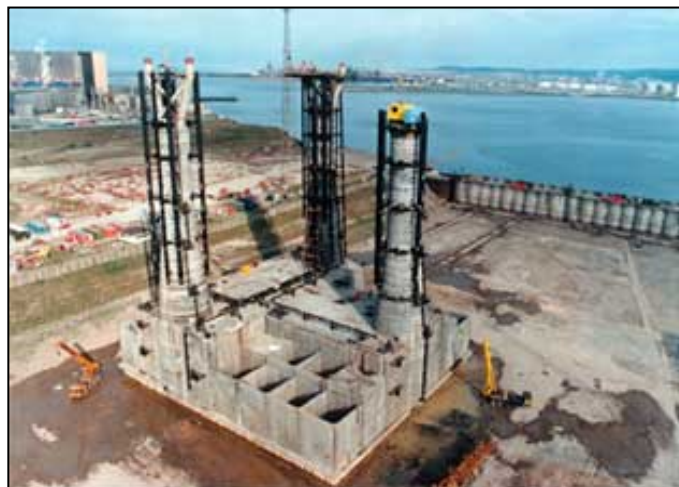
Figure 5-25: GBS Construction in a Dry-dock Facility
