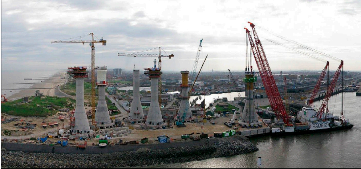
Figure 5-23: Construction of GBS on the Quay (Thornton Bank)
