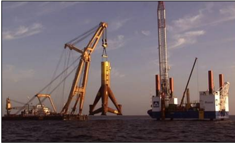
Figure 4-2: Shearleg Crane-vessel Working in Tandem with a Jack-up Piling Vessel
