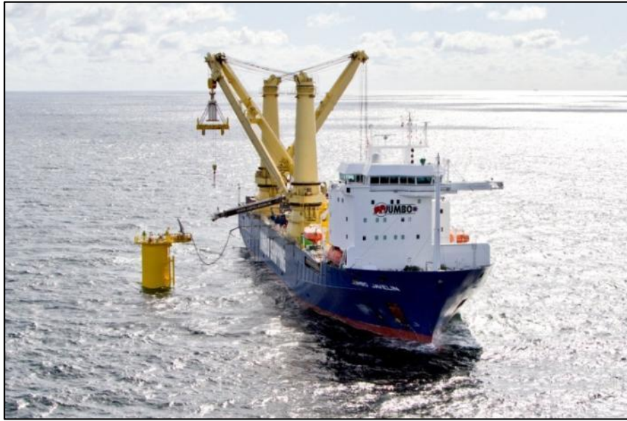
Figure 4-4: Jumbo Javelin Installing Transition Piece, Anholt Offshore Wind Farm, Denmark
