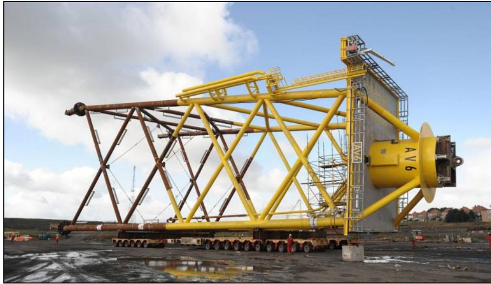
Figure 5-20: Jacket Transportation on the Quay
