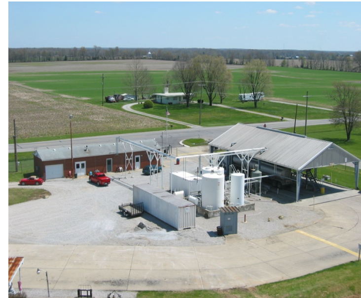
Hartford Woodrider Terminal in Seymour, Indiana installed a 30,000 gal fully automated biodiesel blending system
