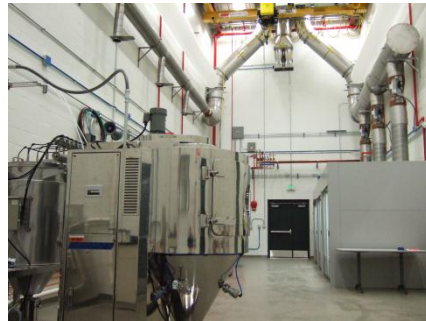
Dry processing area
