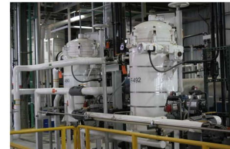
Rockwood lithium hydroxide production
