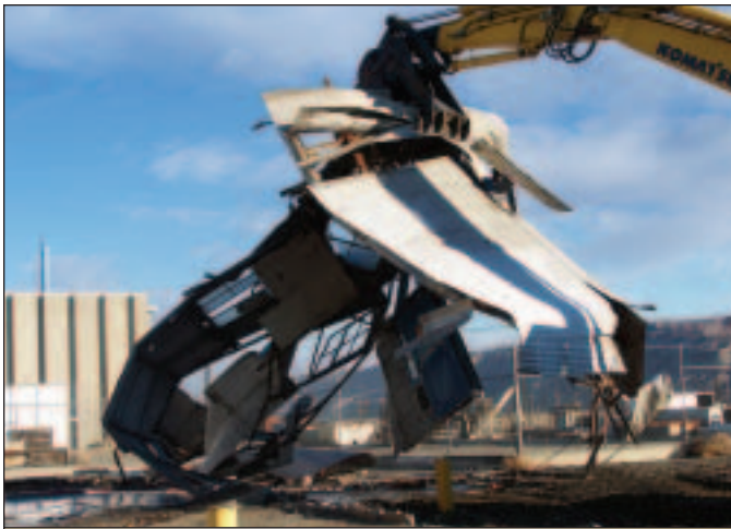
Radioactive Facility Demolition: The demolition of the decontaminated 334A Waste Acid Storage Building at the Hanford Reservation at Richland, Washington.
