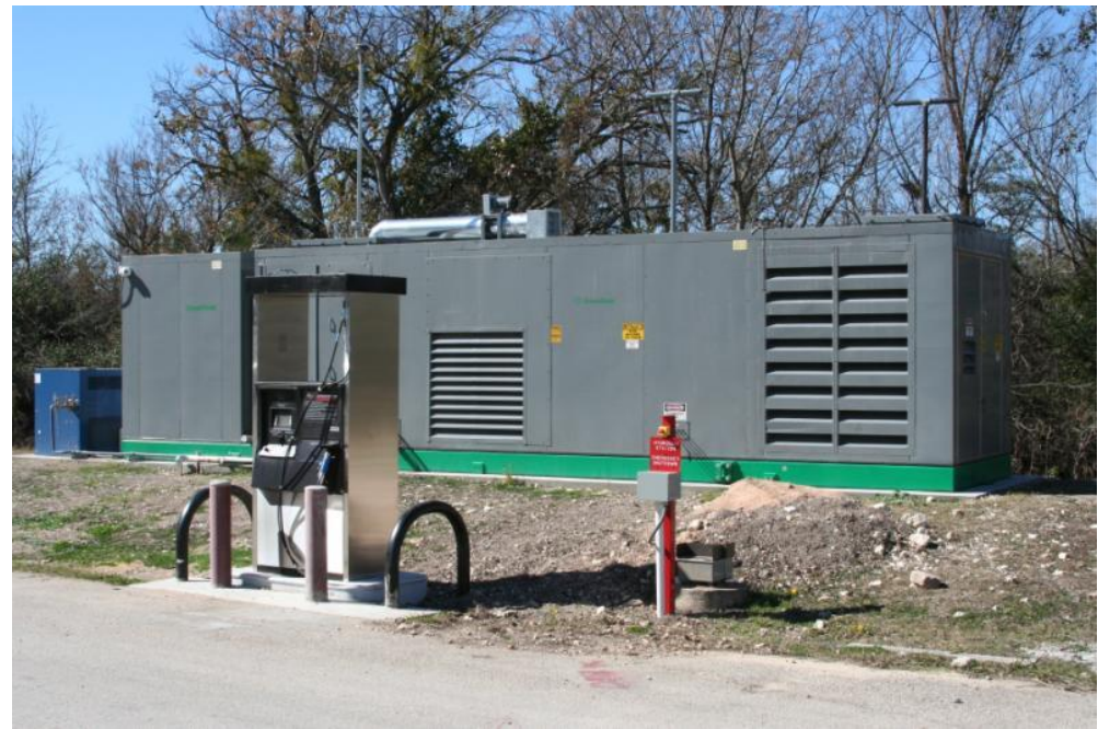
Hydrogen fueling dispenser
