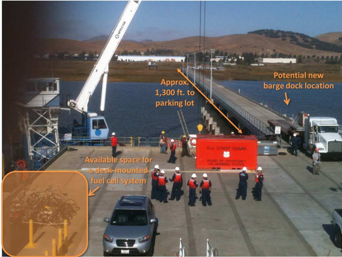
Figure 4-16: SBRF facility, view from the APL looking towards shore.
