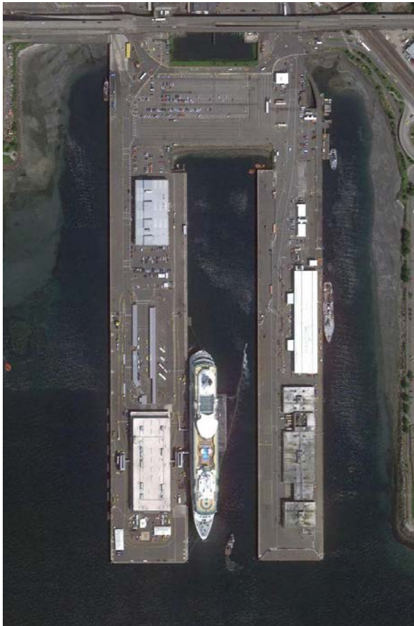
Figure 4-8: Close-up satellite view of Pier 91 at the Port of Seattle (image by Google).
