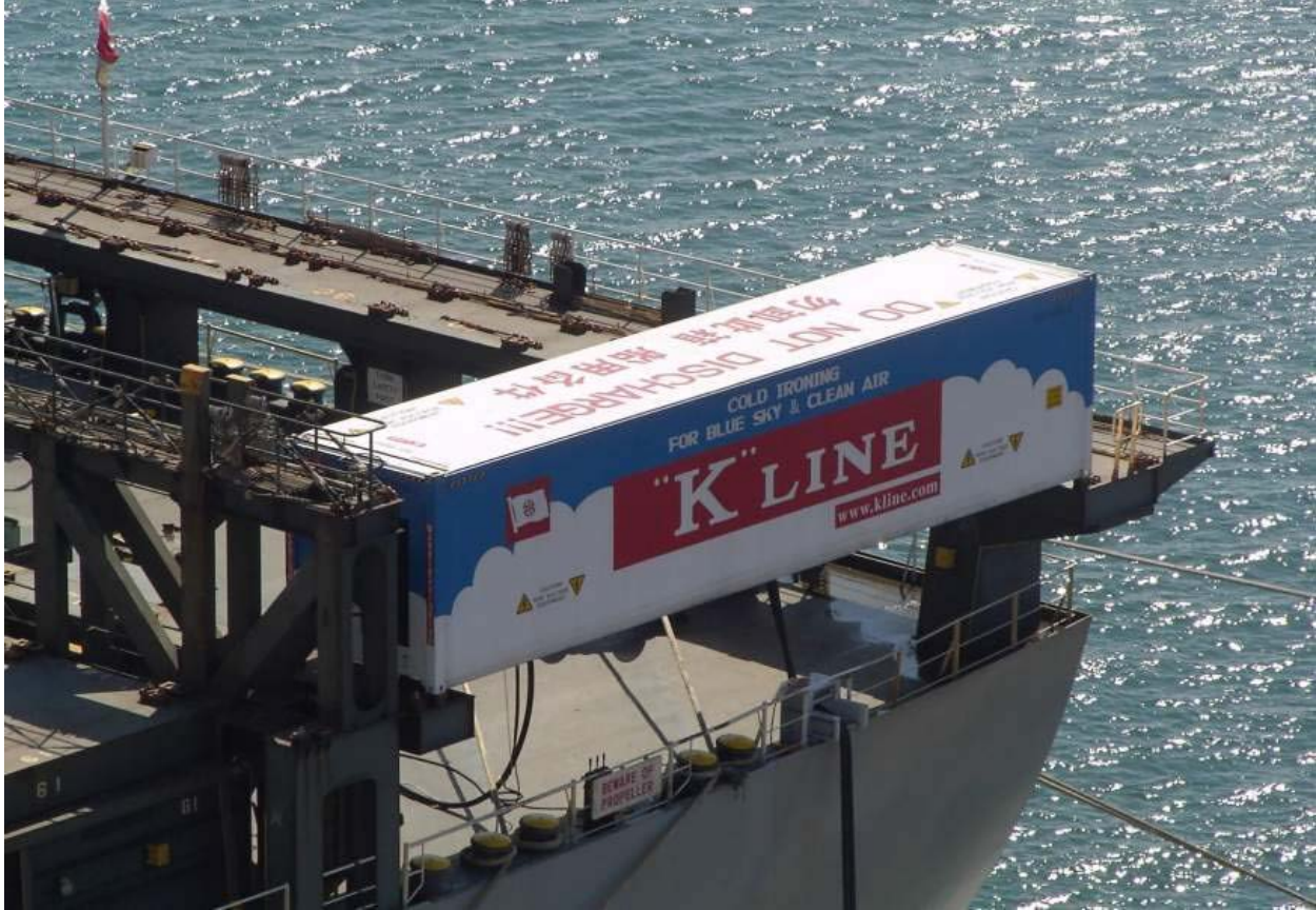
Figure 2-16: The ship-side shore power connection in a specialized shipping container mounted at the stern of one of “K” Line’s five retrofitted container vessels [38].
