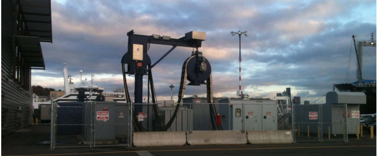
Figure 2-19: Shore power infrastructure for the cruise terminal at Pier 91, Port of Seattle. In this picture, the cable handling system is shown its storage position. During cruise season (May – September) it is moved to the edge of the dock.
