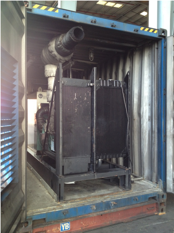
Figure 3-9: A containerized, 300 kW diesel generator with a 1,800 gallon diesel tank, used to provide power for 20-30 reefer containers while on the dock and during transit.
