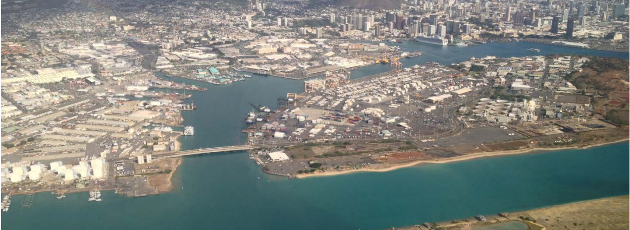
Figure 4-12: Aerial view of Honolulu Harbor. In the foreground is Sand Island, home to the major container terminals. Near the top, middle right a cruise ship at berth can be seen at the cruise terminal.
