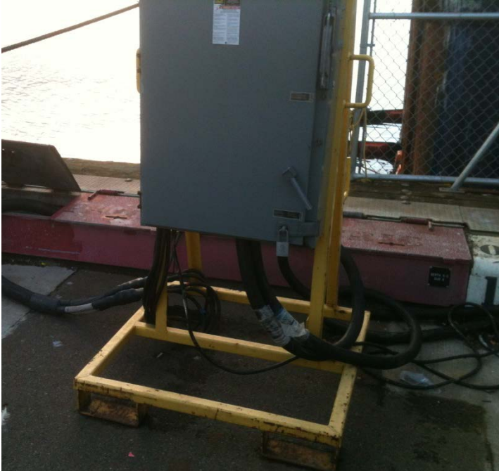
Figure 4-9: Small-vessel shore power disconnect box being utilized by a fishing trawler at the Port of Seattle's Pier 91.
