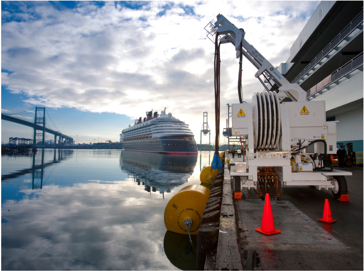
Figure 2-20: An "AMP Mobile" unit at the Port of Los Angeles' World Cruise Center. The Port has three units and is capable of supplying shore power to two cruise ships simultaneously with up to 20 MW of power each [40].
