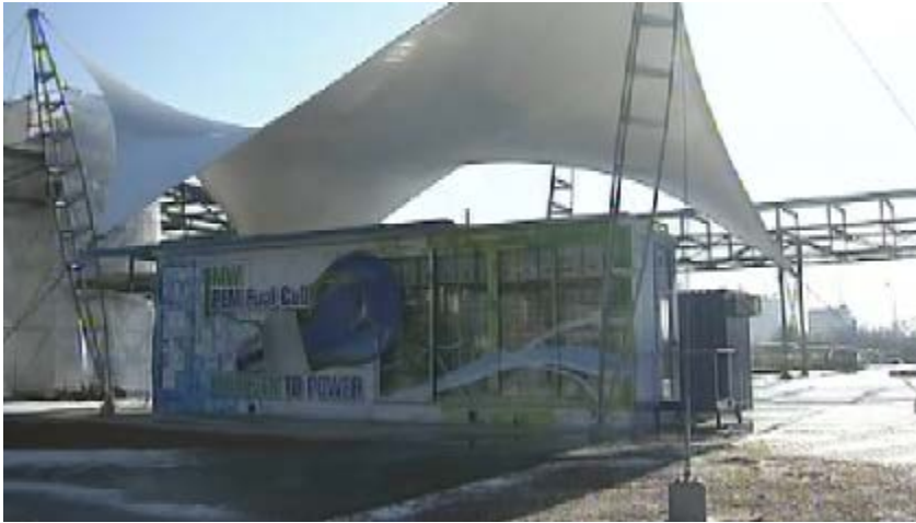
Figure 3-3: A 1 MW PEM system by Nedstack recently installed at a chlorine plant in Antwerp, Belgium [69].
