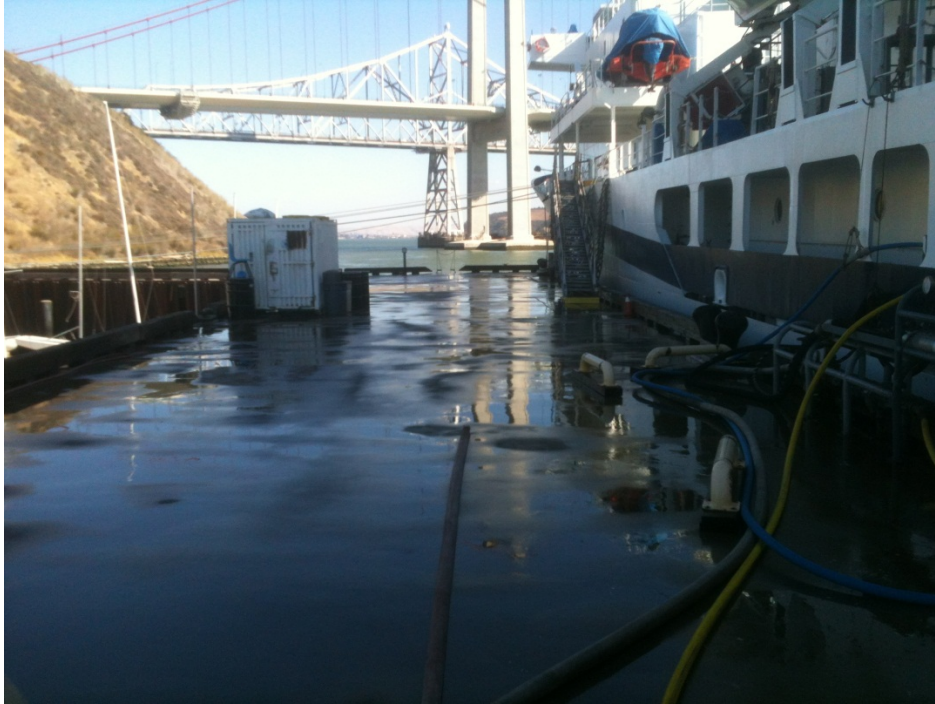
Figure 4-21: The dock area next to the TSGB. The current location of the white container would be the preferred option for a containerized hydrogen-fueled PEM fuel cell system. Electrical tie-in to the vessel is just behind and to the right of the photographer; cables would be run under the dock.
