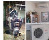
(Left) The original diesel boiler was encapsulated in asbestos, in place to eliminate remediation cost as provide a robust backup heating source in extreme weather. (Right) The new HSPF 9.4, four-head ductless pump system will drastically reduce fuel costs and energy consumption.
