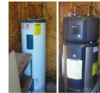
Figures 6-7. Pre-retrofit electric tank water heater, EF = 0.88 (left), hybrid heat pump water heater, COP = 2.35 (right).
