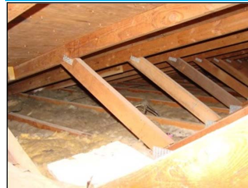
R-38 Ceiling Insulation
