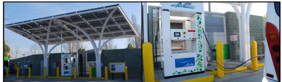
AC Transit fueling station (Photo courtesy of L. Eudy, NREL)
