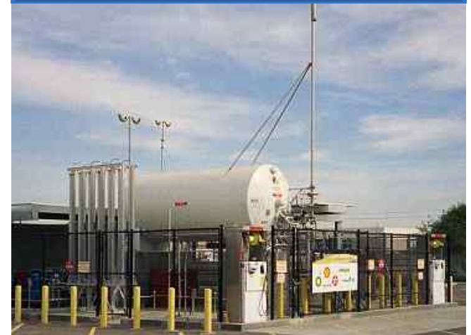
LH 2 Tank/ Fueling Station
