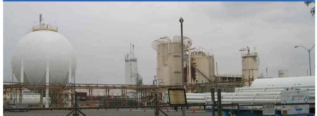
H 2 Plant, Liquefier, LH 2 storage
