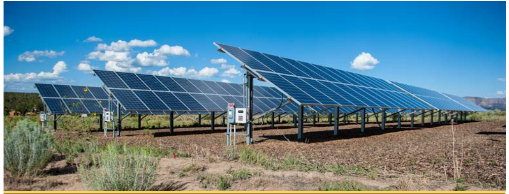
Technical assistance provided through the DOE Office of Indian Energy's START Program is advancing a variety of tribal renewable energy projects, including community- and commercial-scale solar projects. Photo by Dennis Schroeder, NREL 26968
