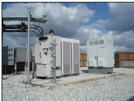
Figure 14: IdaTech Back-up Fuel Cell
