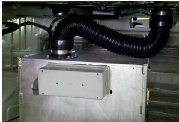
Figure 28. Junction box and the cooling duct.
