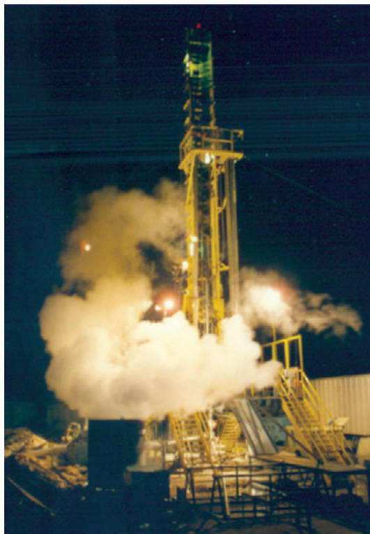
Figure 41. Slimhole production flow test at Steamboat Hills, Nevada
