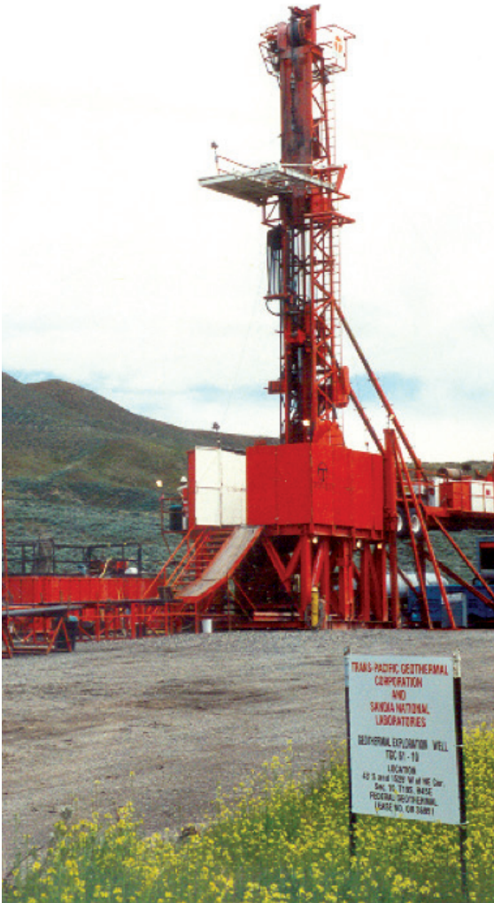
Figure 42. Drill rig at Vale, Oregon
