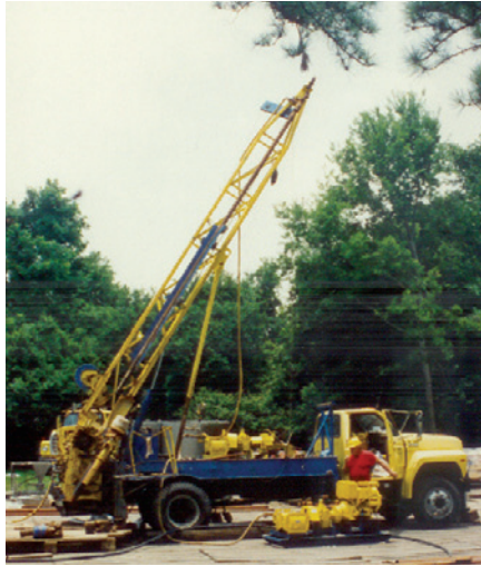
Figure 49. Slant-drilling into the sinkhole at Weeks Island, Louisiana
