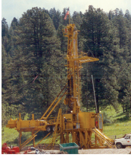
Figure 48. Drilling at VC-2B in northern New Mexico
