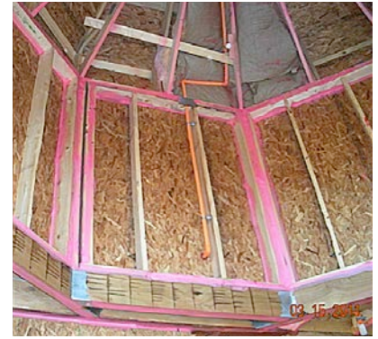
Spray-applied elastomeric air sealing materials simplified air sealing the complex framing design and resulted in tight construction.
