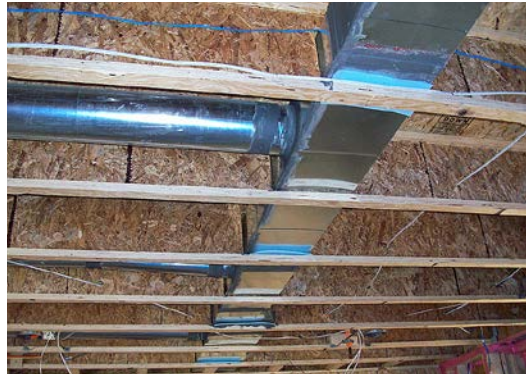
Factory cut floor joists were part of a comprehensive strategy for getting ducts in conditioned space.
