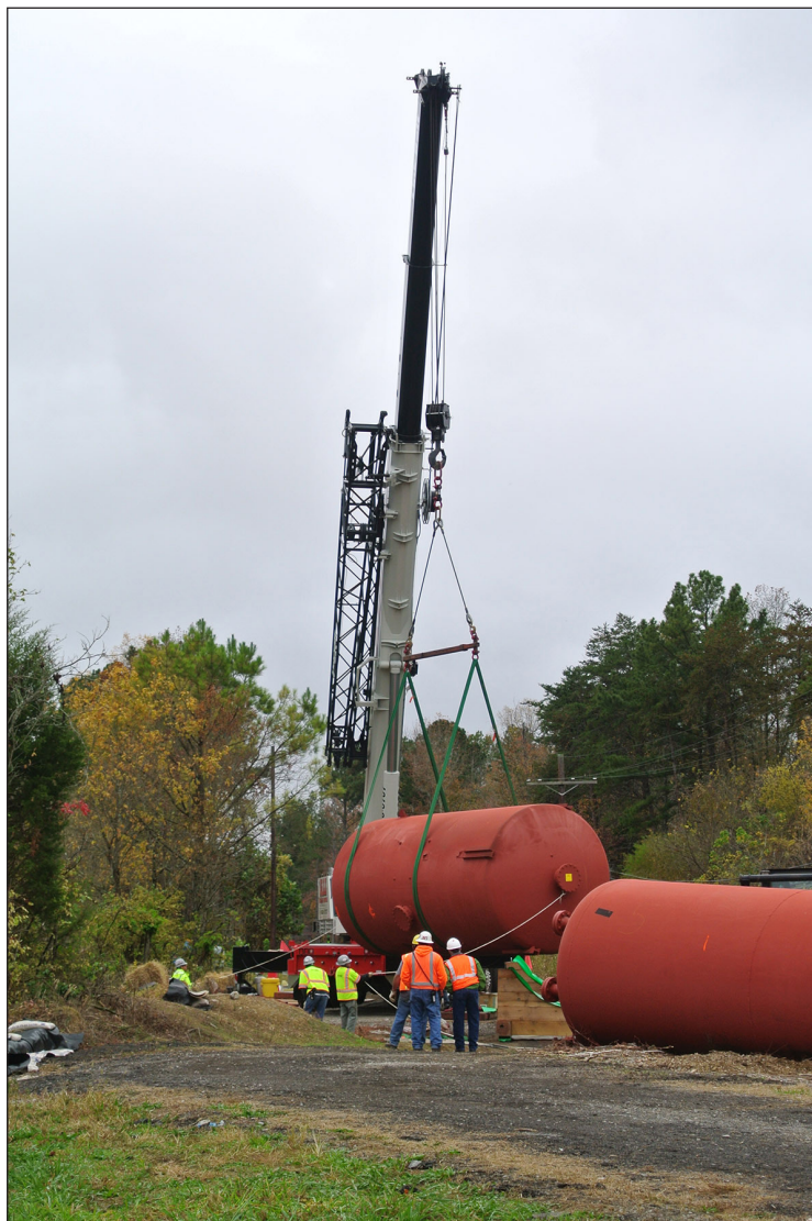
Abandoned tanks at the Y-12 Complex
