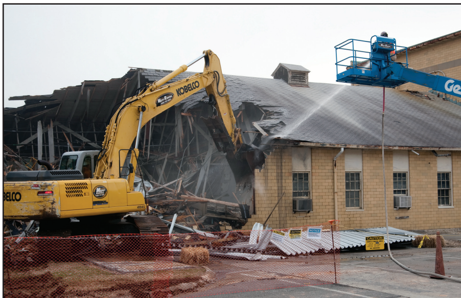
Building 9735 has been demolished.
