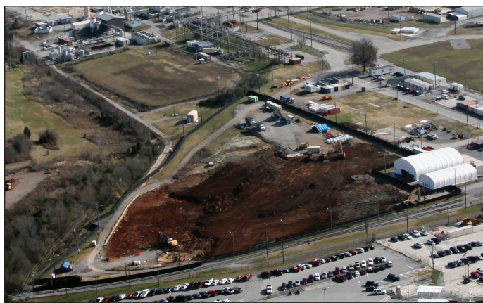
K-1070-B during remediation
