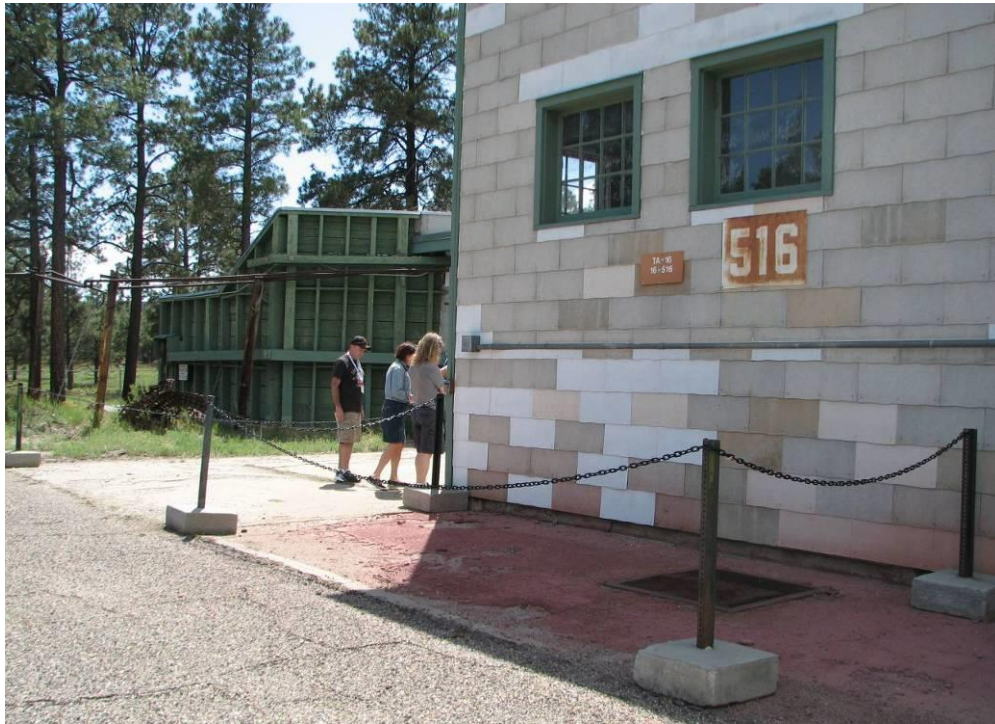
Figure 5. New chain and post barrier protecting the Hubbelite™ work surface.
