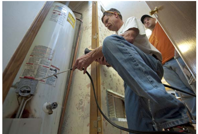
In addition to measuring a water heater's efficiency, an energy assessor also checks carbon monoxide levels in any home scheduled for weatherization.
