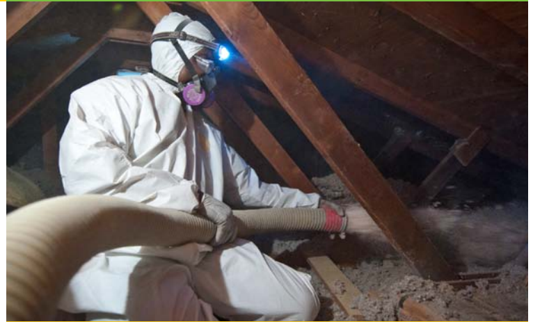
Adding insulation to a home is a typical energy upgrade measure. In this home, a worker blows in cellulose insulation to bring the R value up to R38.
