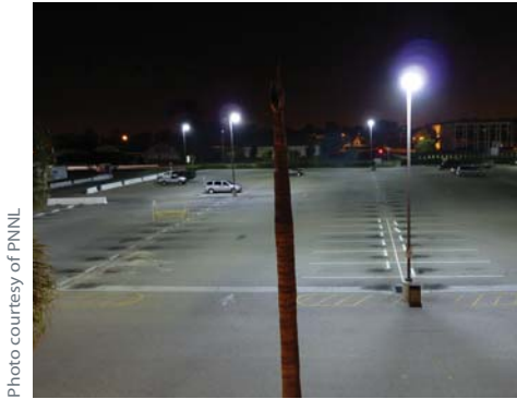
Figure 3: Navy Exchange with new 207-Watt LED lighting system. Note uniformity of LED. Photo taken with a Panasonic DMC-ZS1, 3.2 second exposure, F3.3, June 10, 2010.
