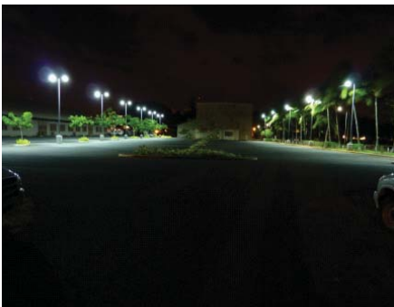
Figure 5: Parking Lot A with new 250-Watt induction lighting system. Photo taken with a Panasonic DMC-ZS1, 4 second exposure, F3.3, June 24, 2010.
