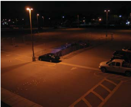
Figure 1: Commissary baseline with 400-Watt high-pressure sodium lighting system. Photo taken with a Canon PowerShot S500, 1/8 second exposure, F2.8, February, 2009.
