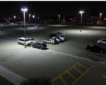
Figure 2: Commissary with new 250-Watt induction lighting system. Photo taken with a Panasonic DMC-ZS1, 1.6 second exposure, F3.3, June 9, 2010.
