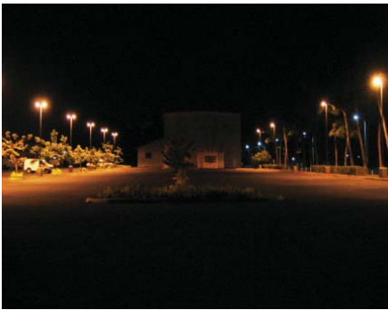
Figure 4: Parking lot A baseline with 400-Watt high-pressure sodium lighting system. Photo taken with a Canon PowerShot S500, 1/8 second exposure, F2.8, May 21, 2009.
