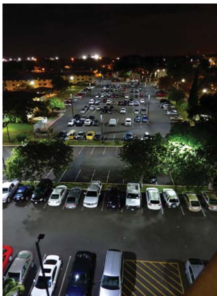
Figure 6: Dormitory Parking Area with new 104-Watt LED lighting system. Photo taken with a Panasonic DMC-ZS1, 4 second exposure, F3.3, June 24, 2010.
