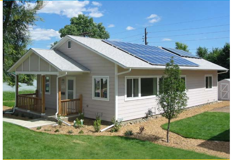
Solar photovoltaic systems are being installed through SERC to reduce clients' energy bills beyond weatherization.
