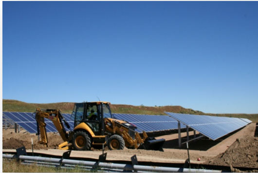
1.7 MW consolidated PV site
