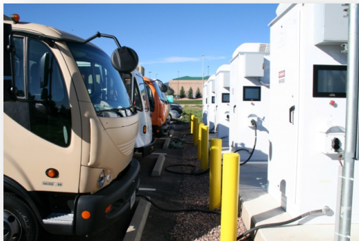
Bi-directional vehicle charging stations
