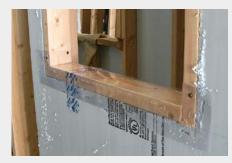
Because the foam is high density, fairly simple window and door framing details can be used. Easily installed plastic sill flashing is an added benefit.
