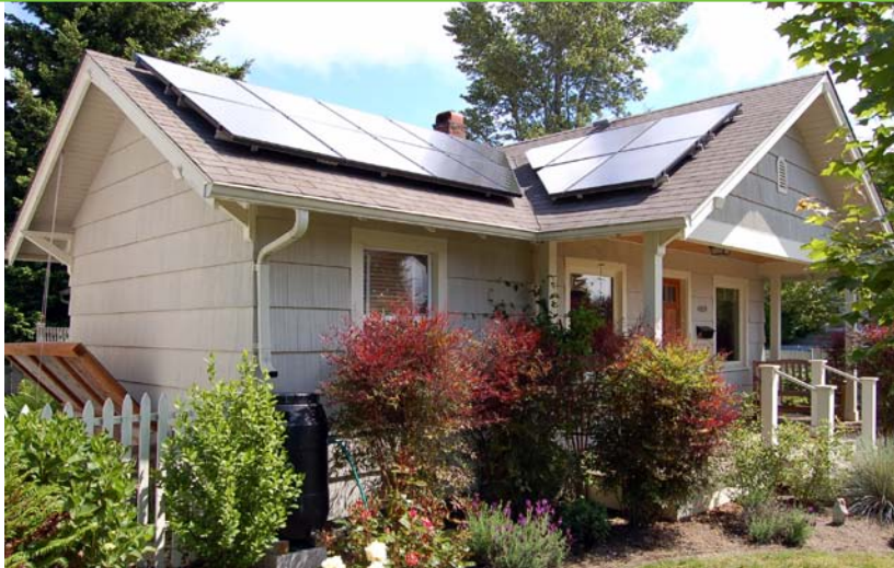
Residential solar installations often face shading issues in tree-friendly Seattle; however, there is often a workable solution. Photo from Brothers Electric, NREL/PIX 19483
