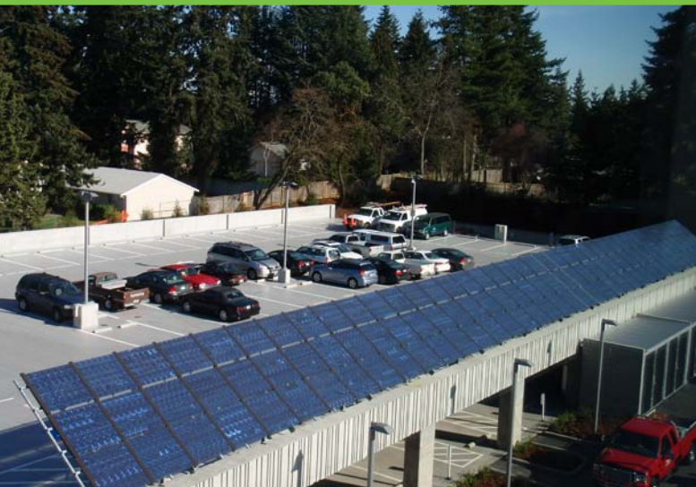
The City of Shoreline, Washington, installed a 20.2-kW solar electric system atop the City Hall parking garage. The system uses made-in-Washington solar modules from Marysville-based Silicon Energy and was installed by Shoreline-based Northwest Mechanical. Shoreline, just north of Seattle, is served by Seattle City Light. Photo from City of Seattle, NREL/PIX 18074
