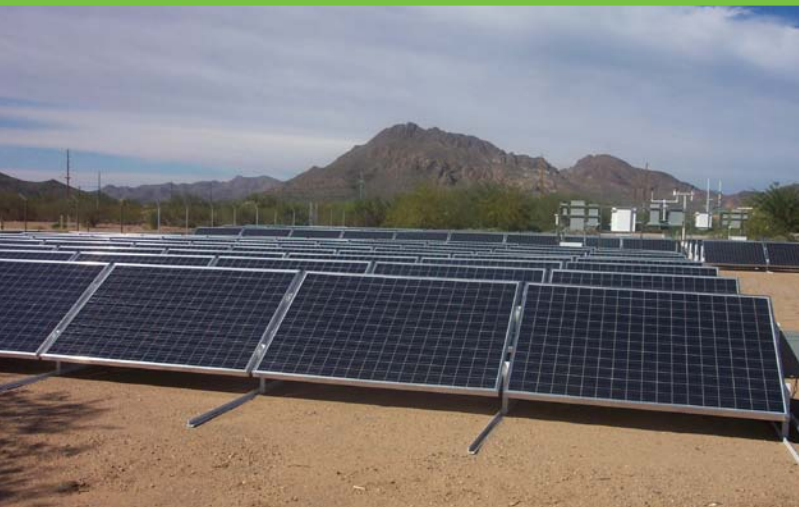
The Hayden-Udall Water Treatment Facility phase I array is the first City of Tucson solar project to take advantage of the many large parcels of land in the metropolitan area. Photo from The City of Tucson, NREL/PIX 18373
