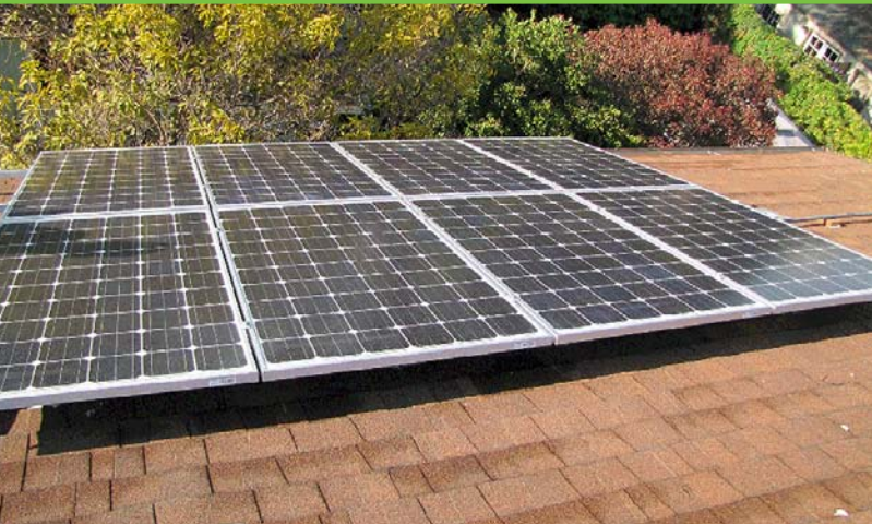
Residential solar systems, such as this 1.7-kW PV array in San Diego, have increased through the Solar America Cities effort. Photo from SunCraft Solar, Inc., NREL/PIX18428
