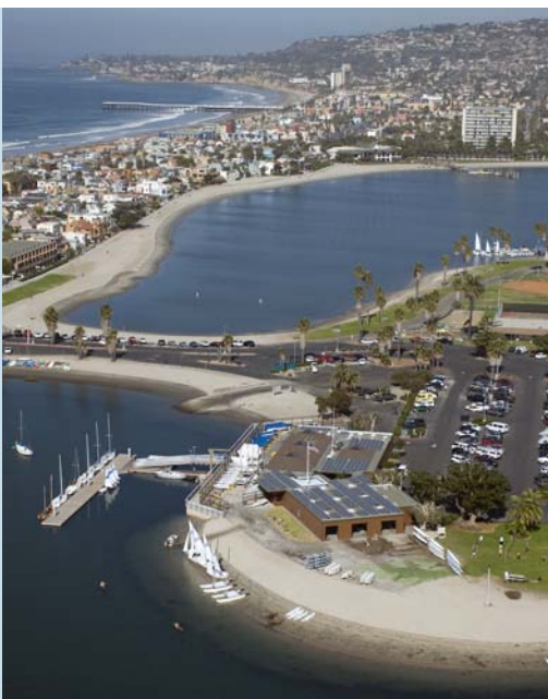
A 40.7-kW PV rooftop installation at the Mission Bay Aquatic Center is shown in this aerial view of San Diego. Photo from Sullivan Solar Power, NREL/PIX 18425
