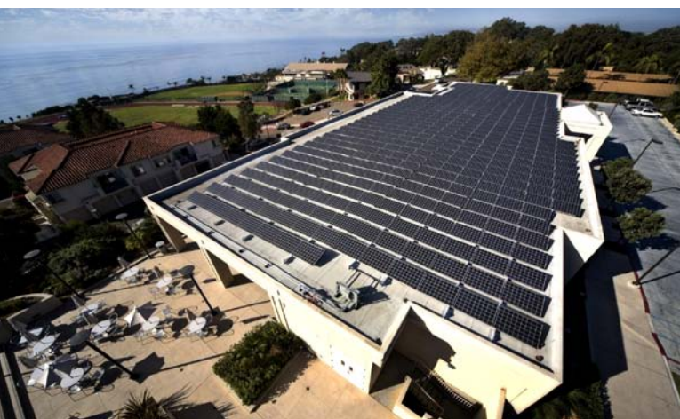
An aerial view of a PV rooftop installation on Point Loma Nazarene University. Photo from SPG Solar, NREL/PIX 18427
