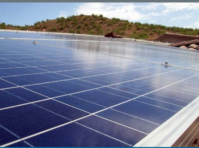
A 6.8-kW photovoltaic installation in San Diego. Photo by Scott Weber, NREL/PIX 18426
