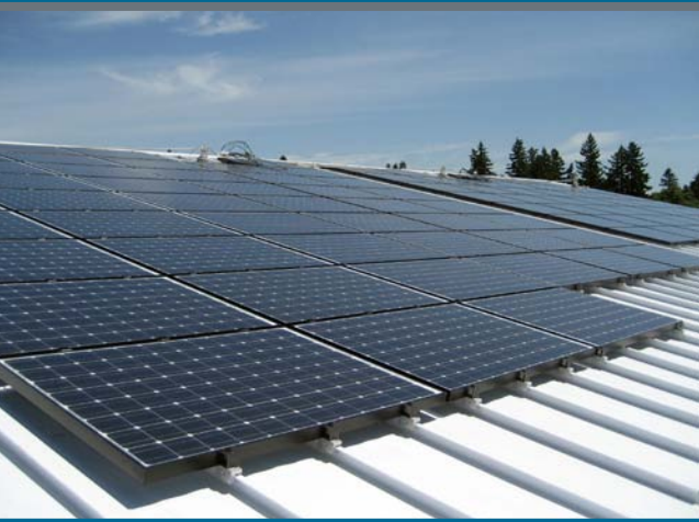
The East Portland Community Center's 87-kW photovoltaic system was installed under a Power Purchase Agreement. Photo from Commercial Solar Ventures, NREL/PIX 18429
