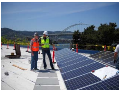
This 12-kW PV array is the largest system entirely owned by the City of Portland. Photo from City of Portland, NREL/PIX 18048
