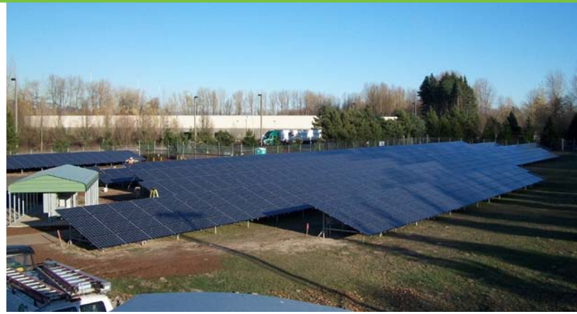
Portland's Columbia Ground Water Pump Station features a 270-kilowatt ground-mounted PV system. Photo from Portland Water Bureau, NREL/PIX 18450
