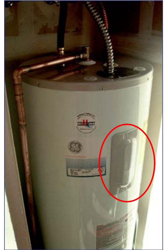
Electric Storage Tank
