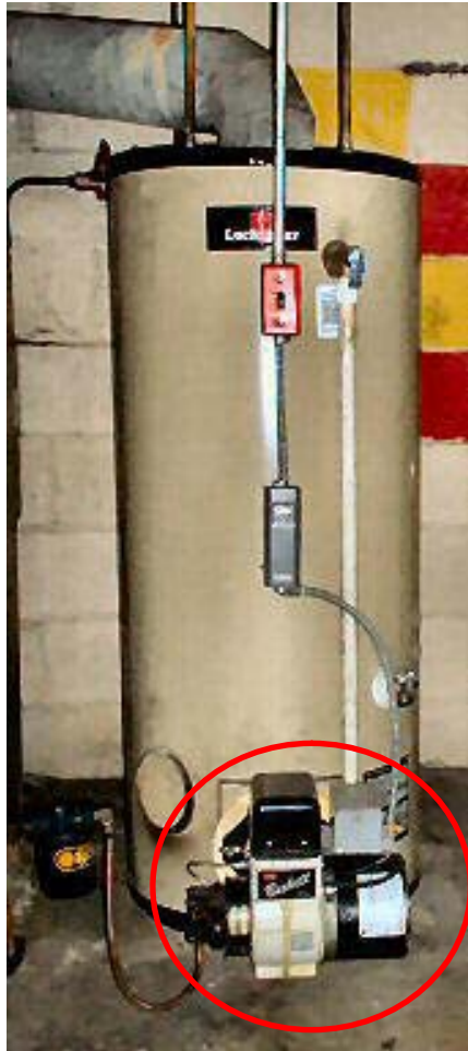
Oil-Fired Storage Tank
