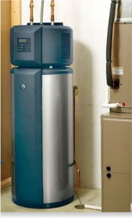
New Heat Pump Water Heater
