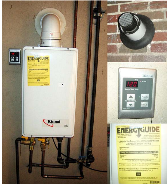
Gas-Fired, Directly Vented, Instantaneous Water Heater
