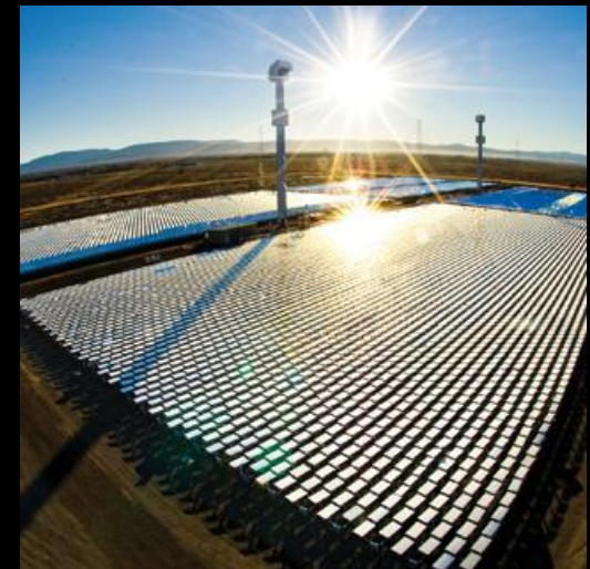
Sierra Project, Lancaster, CA
