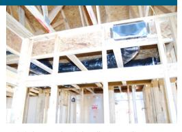
Artistic locates the air handler in a utility room and ducts in a dropped hallway ceiling to protect them from temperature extremes in the attic.
