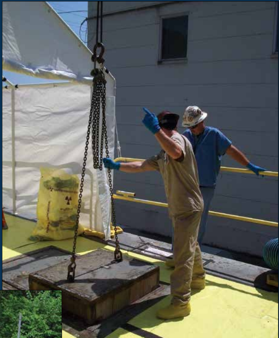
A HEPA shield plug is being removed from a filter pit
