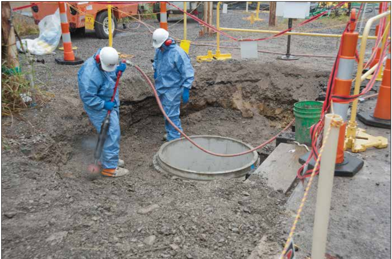
Workers are installing a new catch basin at Y-12 to improve drainage and reduce mercury infiltration
