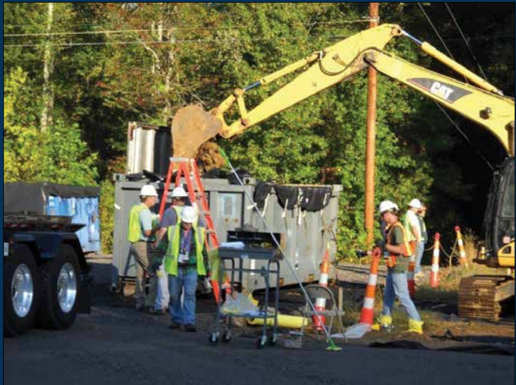
TWPC workers excavate soil for preparation of the sludge test area site
