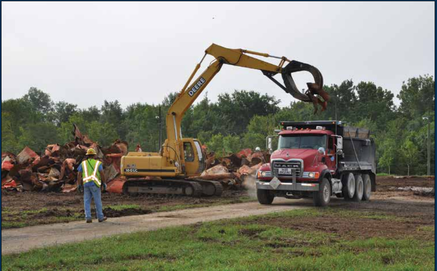
Water tower debris being shipped for disposal
