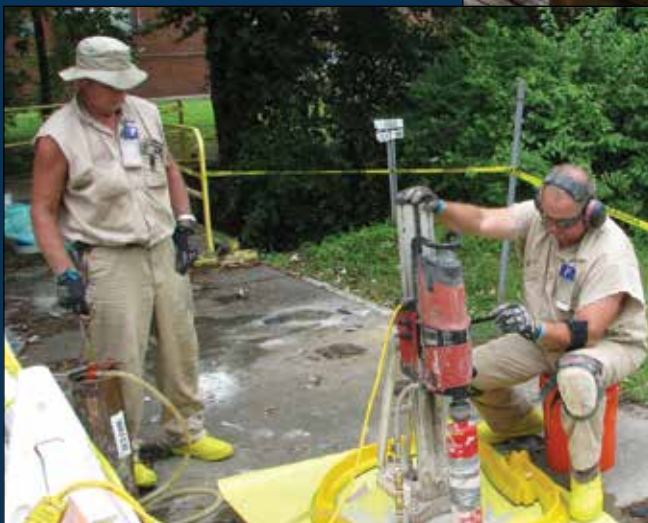
Workers core bore a vent duct cover as part of the 4500 Area gaseous waste system upgrades
