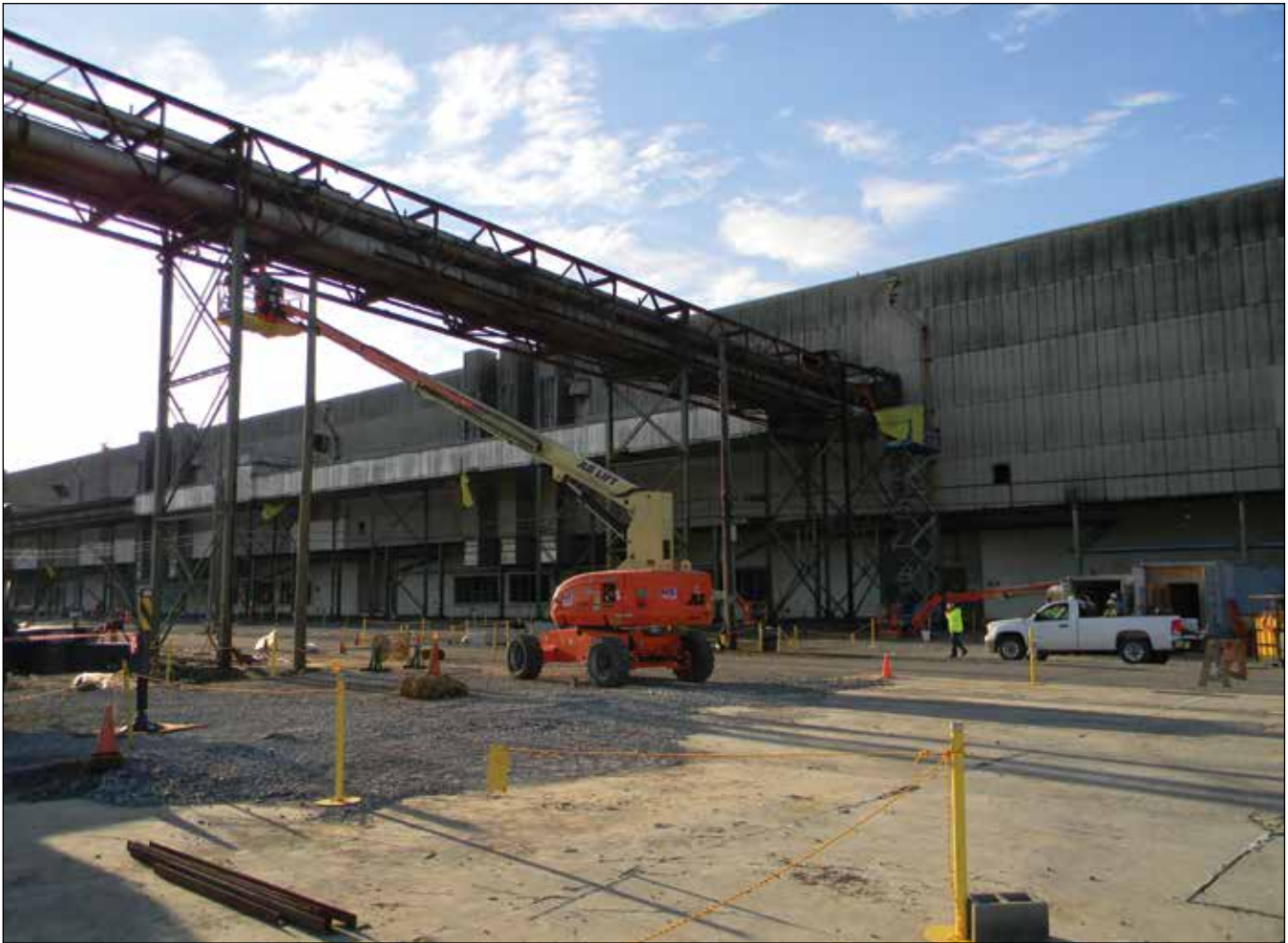
Removal of tie lines that connected K-33 to K-31 marks the completion of the K-33 Building cleanup work
