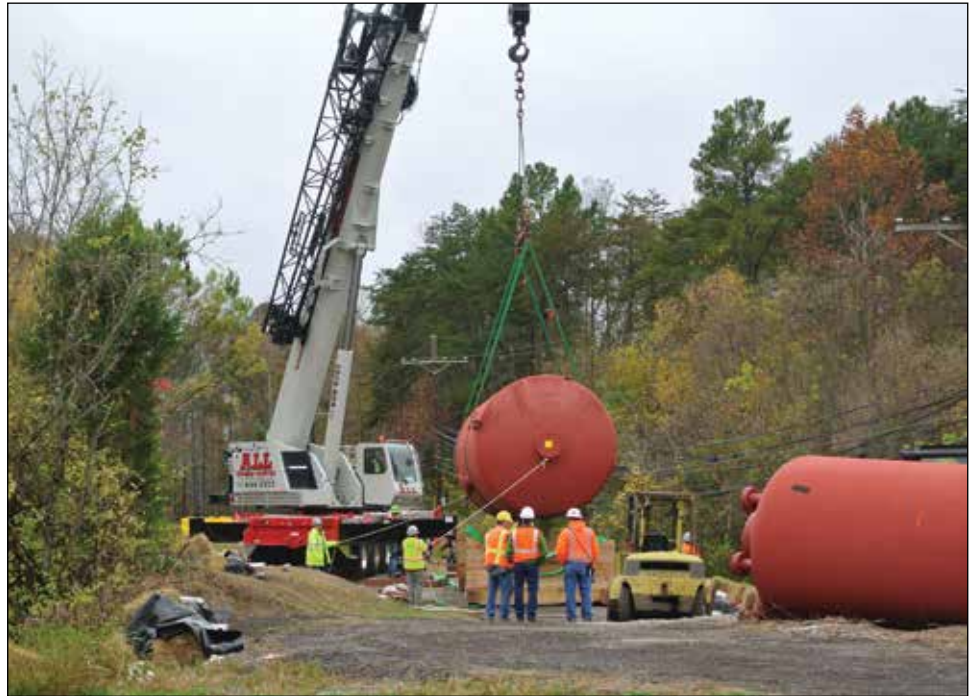
Workers load a mercury-contaminated tank onto an inspection saddle
