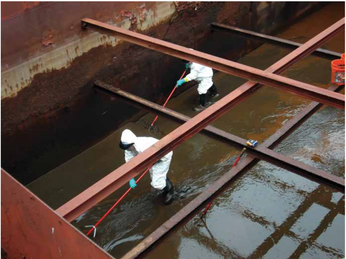
Workers remove sludge from the Central Neutralization Facility as part of the shutdown operations
