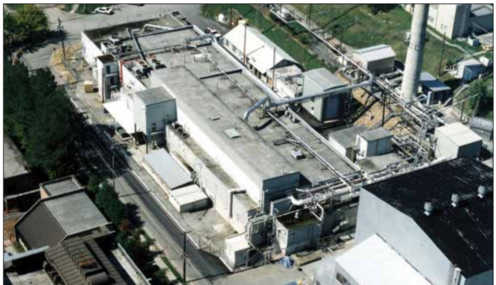
Building 3019A at ORNL
