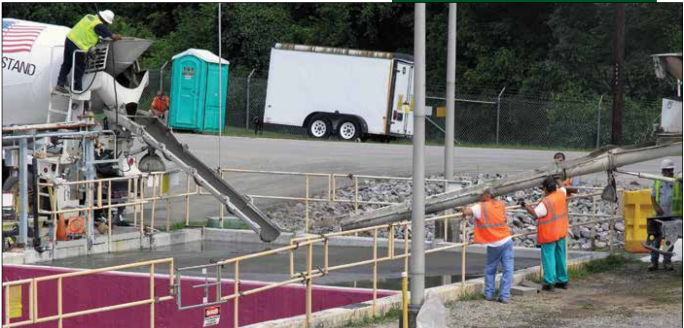
Workers are filling a sump at the TSCA Incinerator
