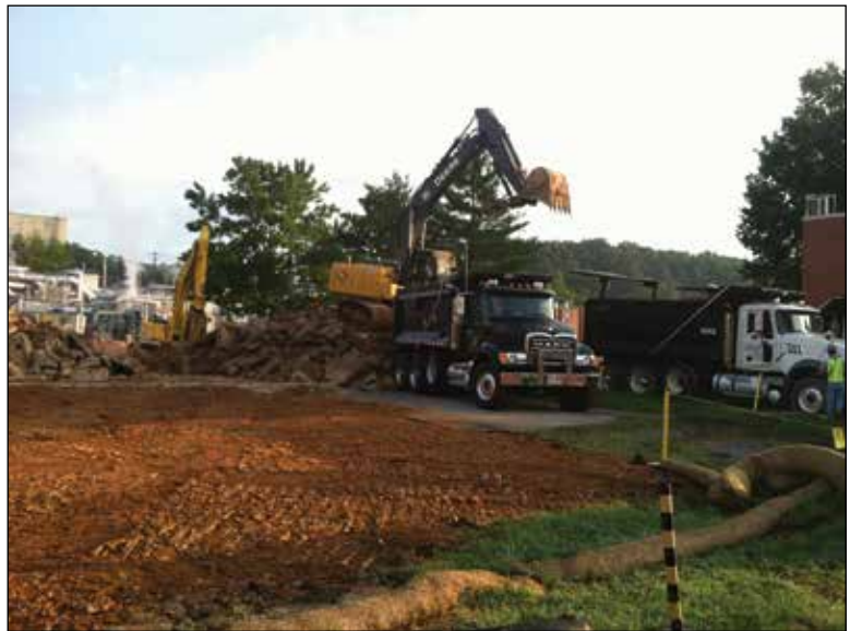
Removal of slab debris at Building 3550 site
