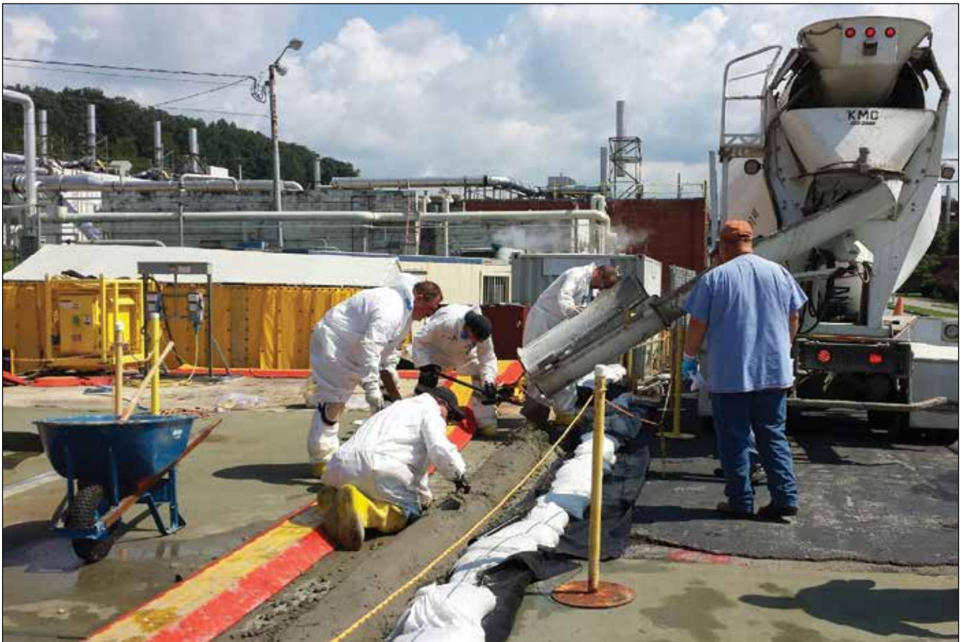
A concrete berm is being poured as part of the 3026 stabilization activities
