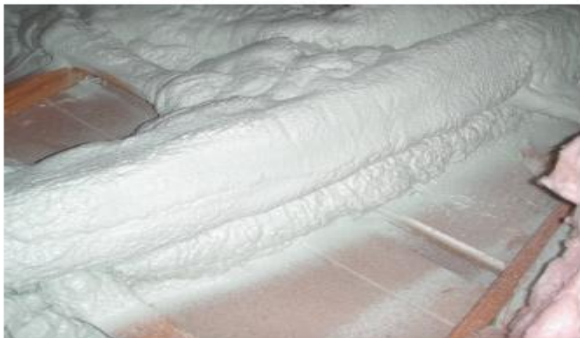
Figure 20. Ductwork well-sealed to sheetrock with ccSPF
