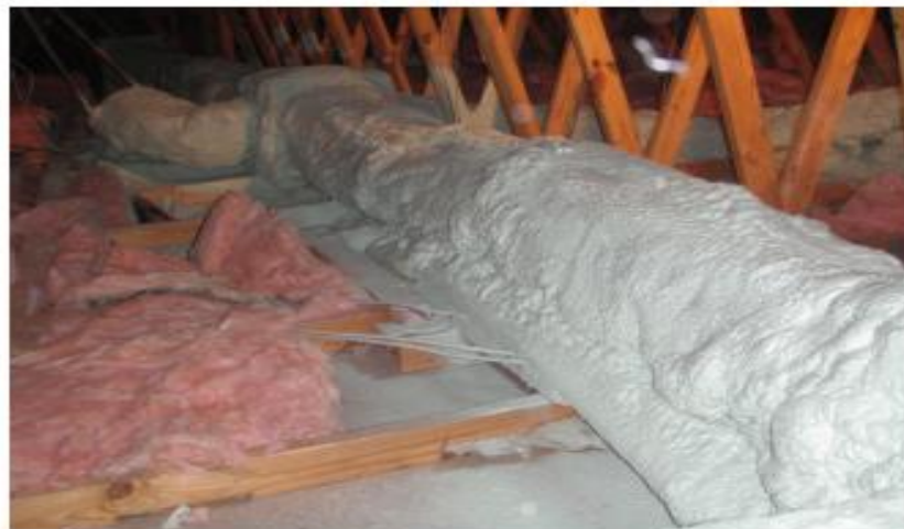
Figure 21. Rigid insulation inserted under ductwork to serve as a substrate and provide insulating value
