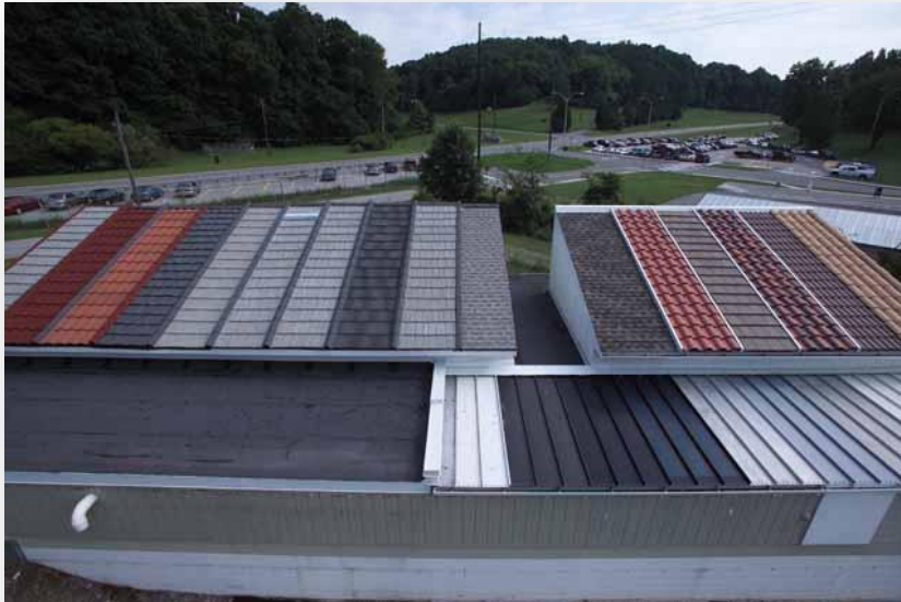
Roof Testing Facility at ORNL Building Technologies Research and Integration Center
