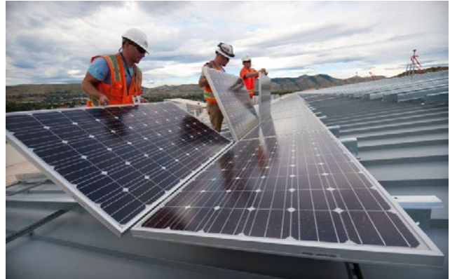
Roof-mounted solar panels help the Research Support Facility reduce its carbon footprint.
