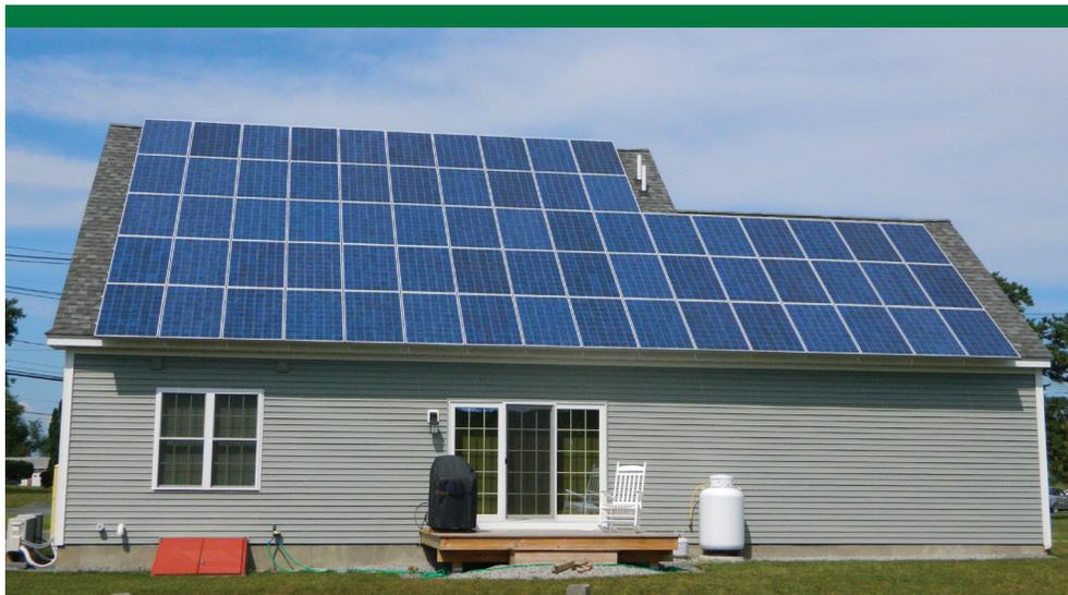
The 68 240-watt solar panels (16.31-kW system) on the south-facing back roof of this production home helped the home achieve a HERS score of -37 and produce more than enough power for this tightly air-sealed (1.26 ACH 50), highly insulated (R-67 attic, R-46 double-wall construction) home.
