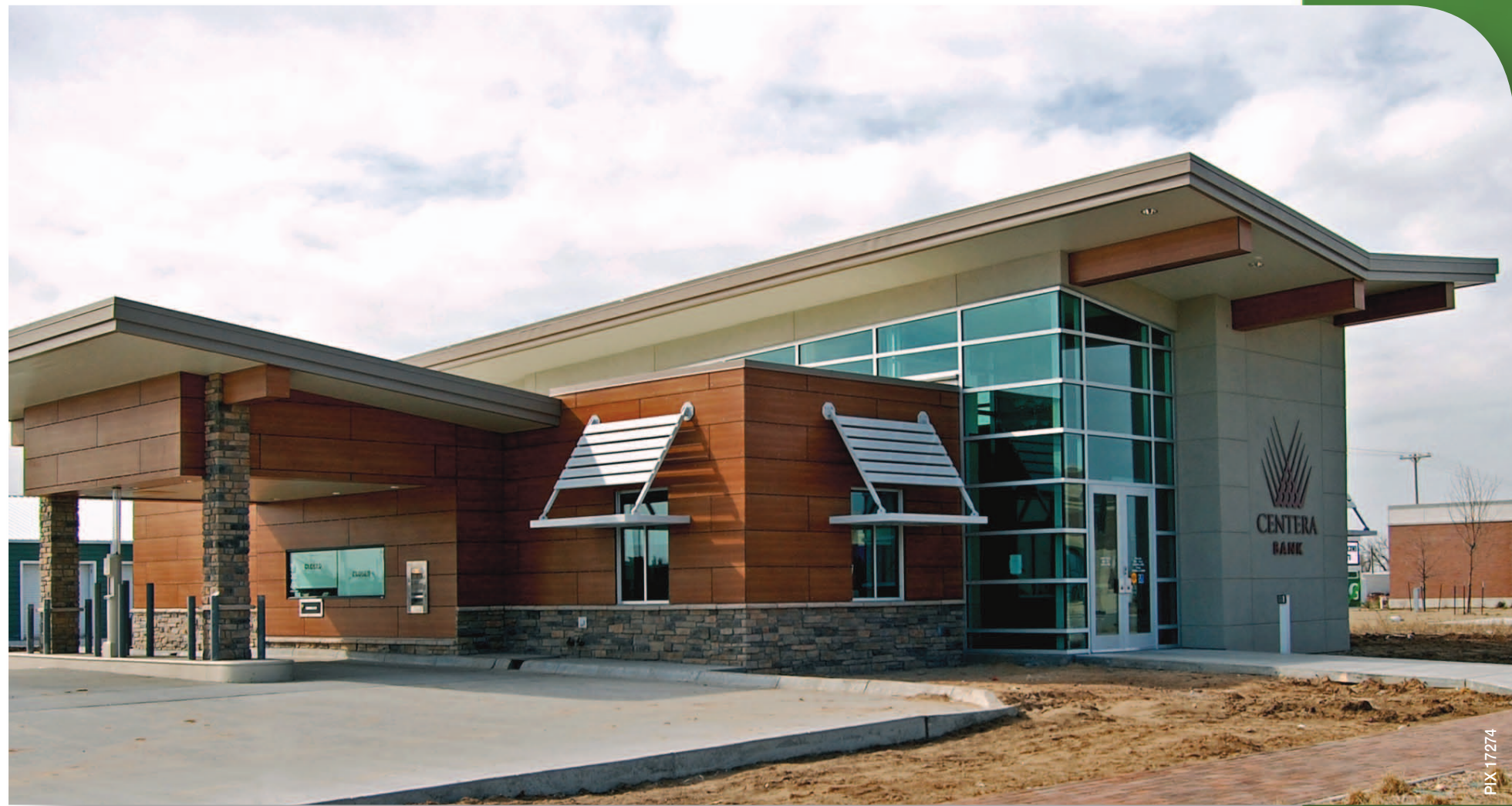
Courtesy of Joah Bussert, Greensburg GreenTown
