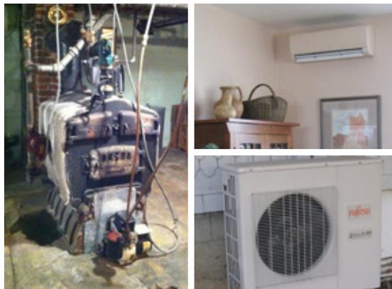
(Left) The original diesel boiler, encapsulated in asbestos, was left in place to eliminate removal and asbestos remediation costs, as well as provide a robust supplemental heating source in extremely cold weather. (Right) The new SEER 16, HSPF 9.4, four-head ductless heat pump system will drastically reduce fuel costs and energy consumption.
