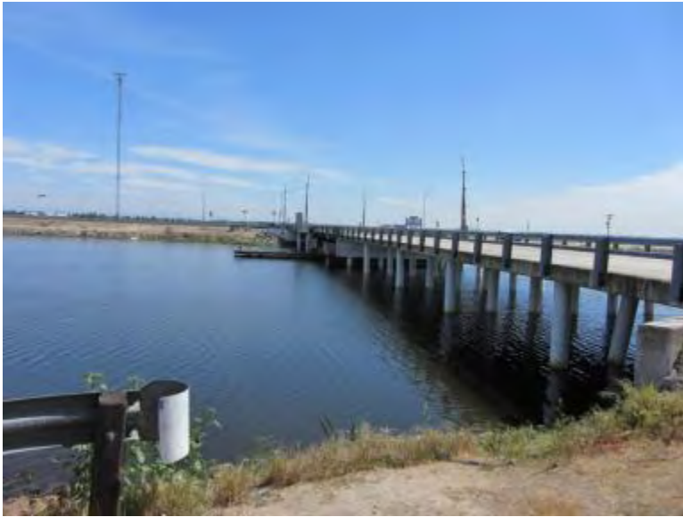
Photograph 9. Bishop Cut at Eight Mile Road Bridge. Swallow nests are present under the bridge. Photograph taken April 3, 2013.
