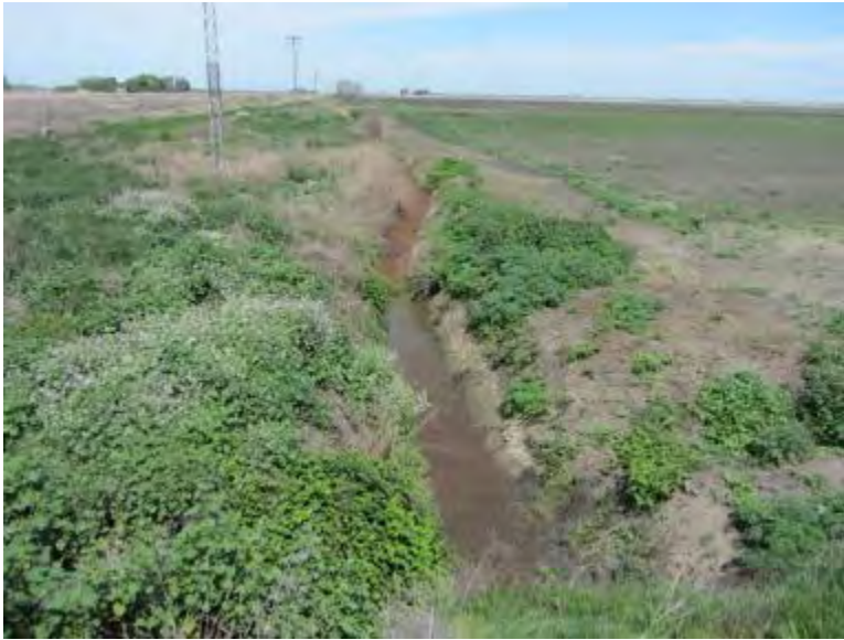
Photograph 11. Representative intermittent irrigation ditch. Ditch located in the eastern pull location work area. Photograph taken April 3, 2013.
