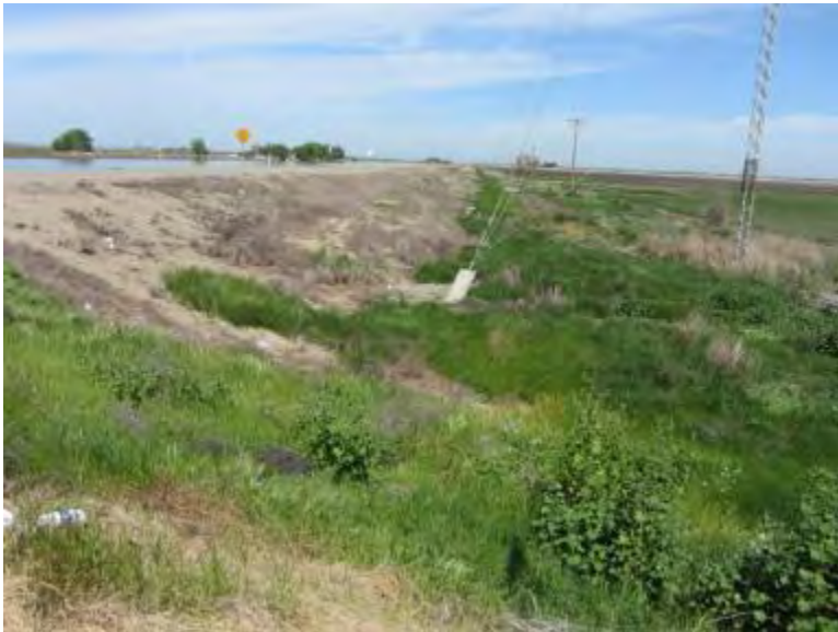
Photograph 10. Eastern pull location and work area at the intersection of King Island Road and Eight Mile Road. Photograph taken April 3, 2013.
