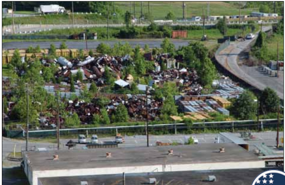
Old Salvage Yard East before scrap removal
