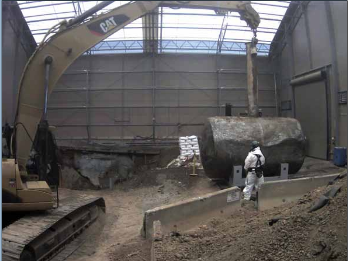
Removal of Tank W-1A at ORNL eliminated the main source of groundwater contamination at the site
