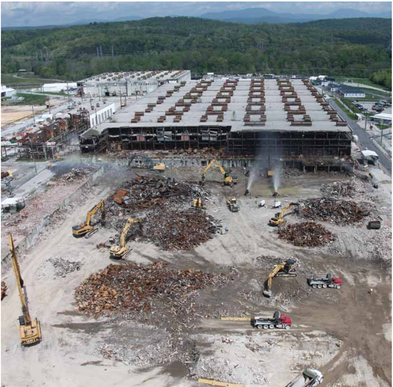
Debris generated from the K-25 demolition project was shipped for disposal as it was generated, with most being disposed of at the Oak Ridge Reservation's Environmental Management Waste Management Facility
