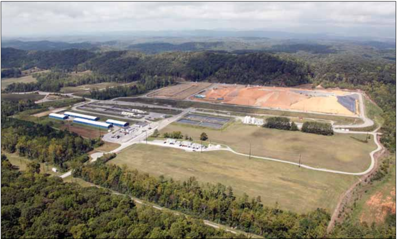
Environmental Management Waste Management Facility
