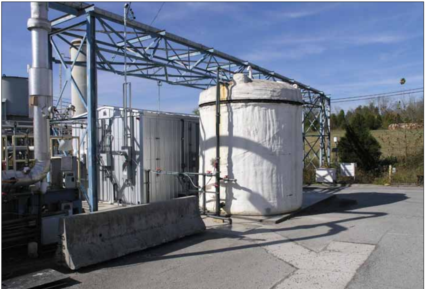
Chromium Water Treatment System
