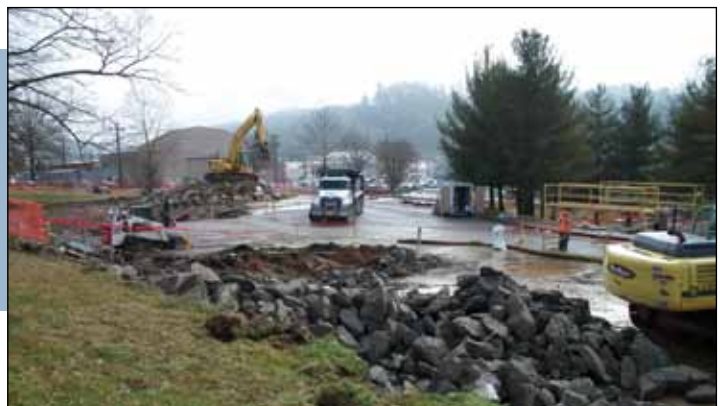
Workers are remediating the Building 2009 and 2010 slab areas
