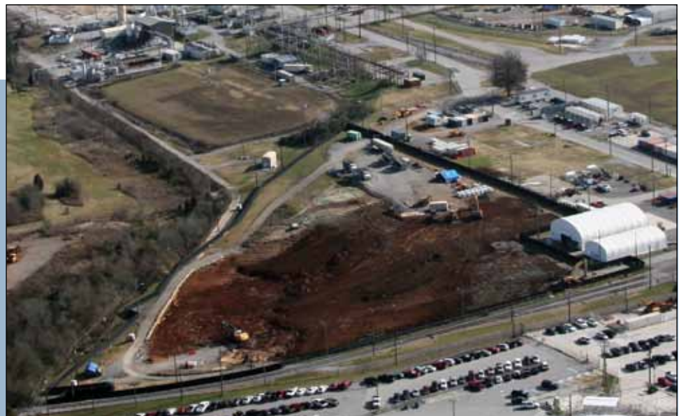
K-1070-B remediation activities
