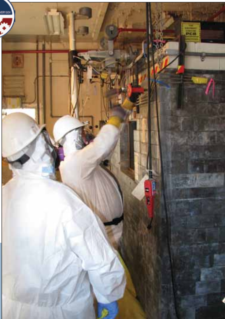
Workers remove lead bricks in the Building 3030 hot cell
