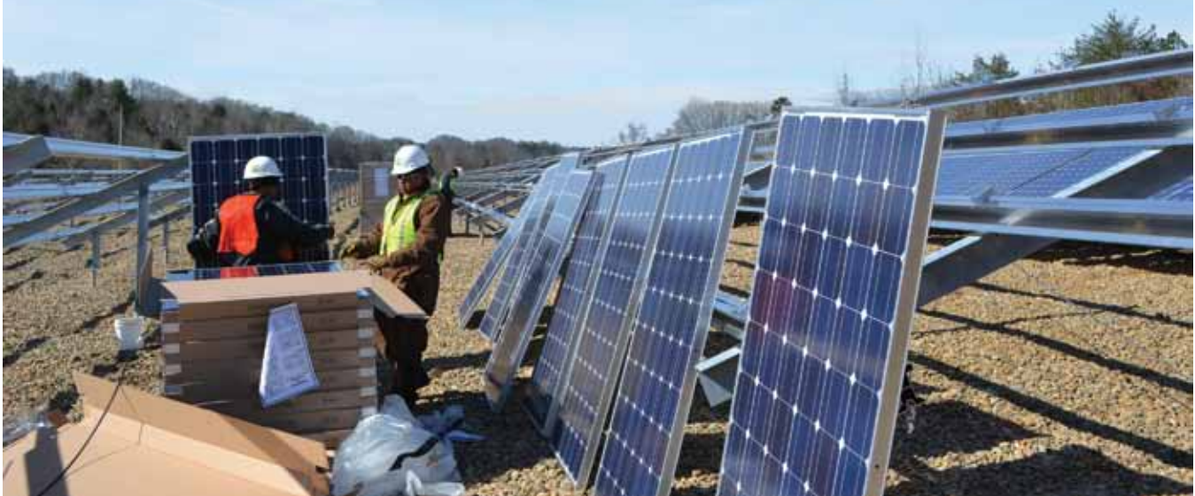
Workers install panels for the solar farm near the ETP entrance
