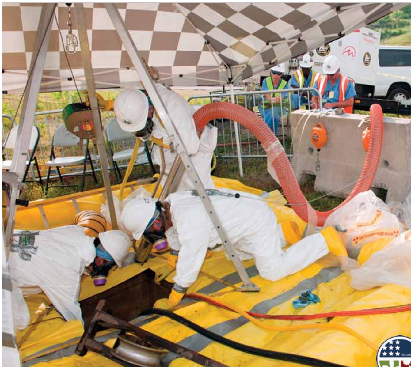
Personnel prepare to insert a vacuum line into the storm sewer basin
