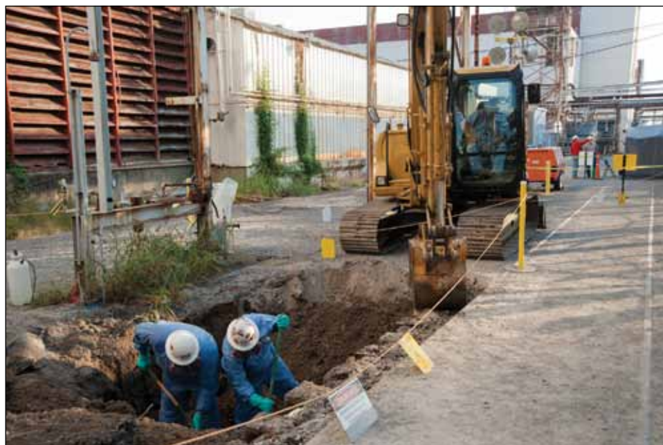
Workers excavate prior to placement of a new storm sewer catch basin behind 9201-5
