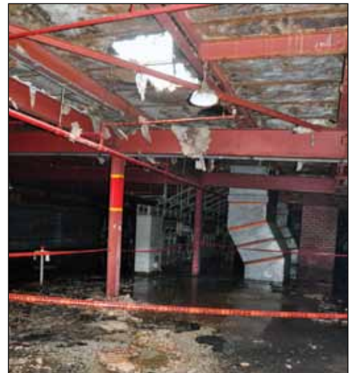
Inside the K-27 Building
