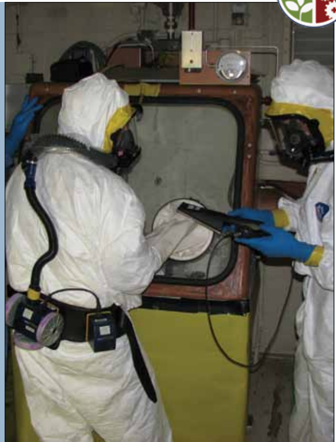
At left, workers are installing a new exhaust duct on the Building 4507 hot cells, and above, workers are stabilizing a glovebox in the building.
