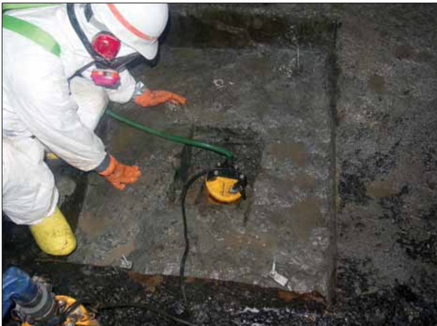
A junction box floor is being prepared to receive a mercury trap
