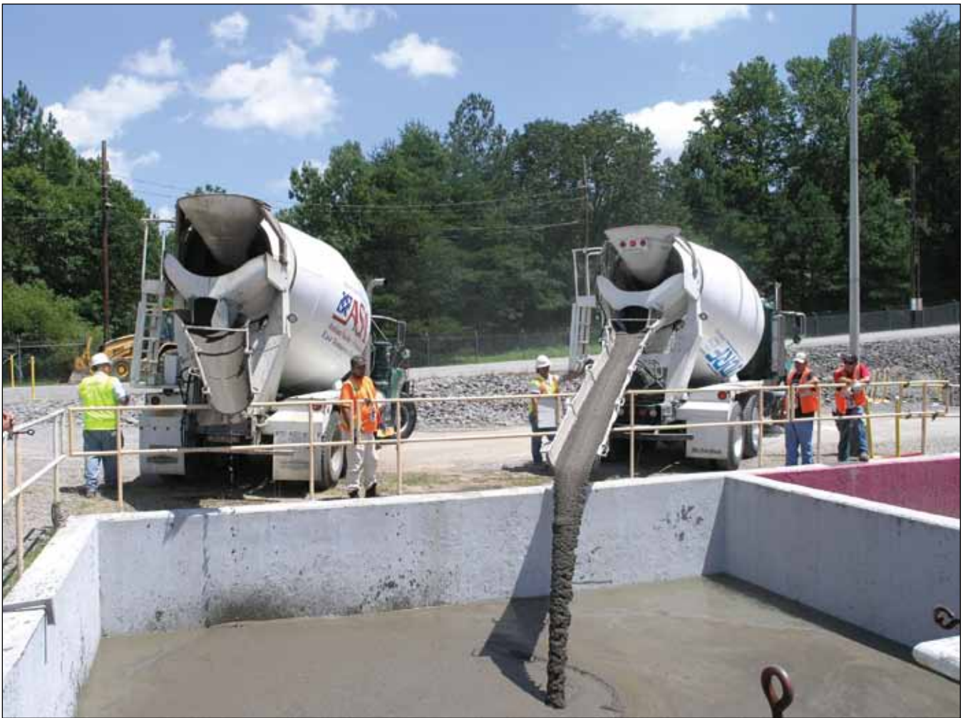
Workers are filling a sump at the TSCA Incinerator
