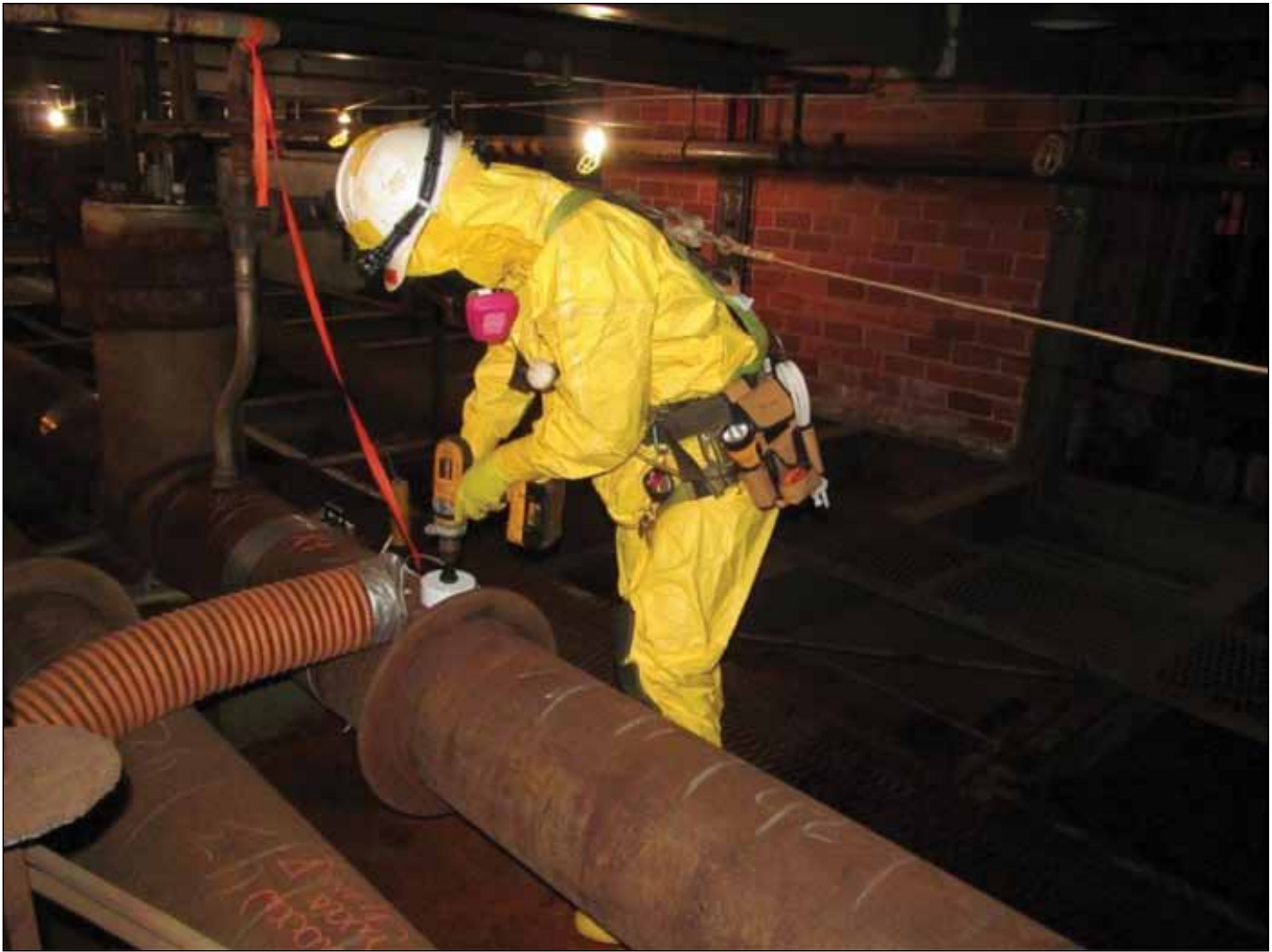
A worker drills a hole in the process gas system piping in K-27 as part of the sampling process
