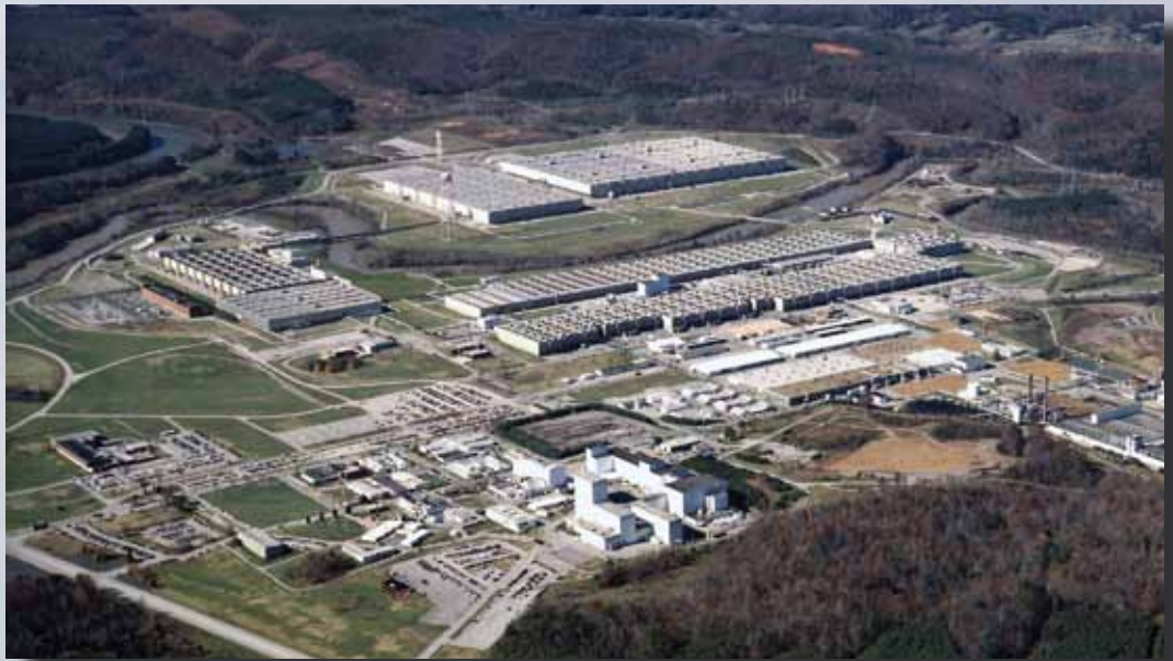
ETTP before cleanup began
