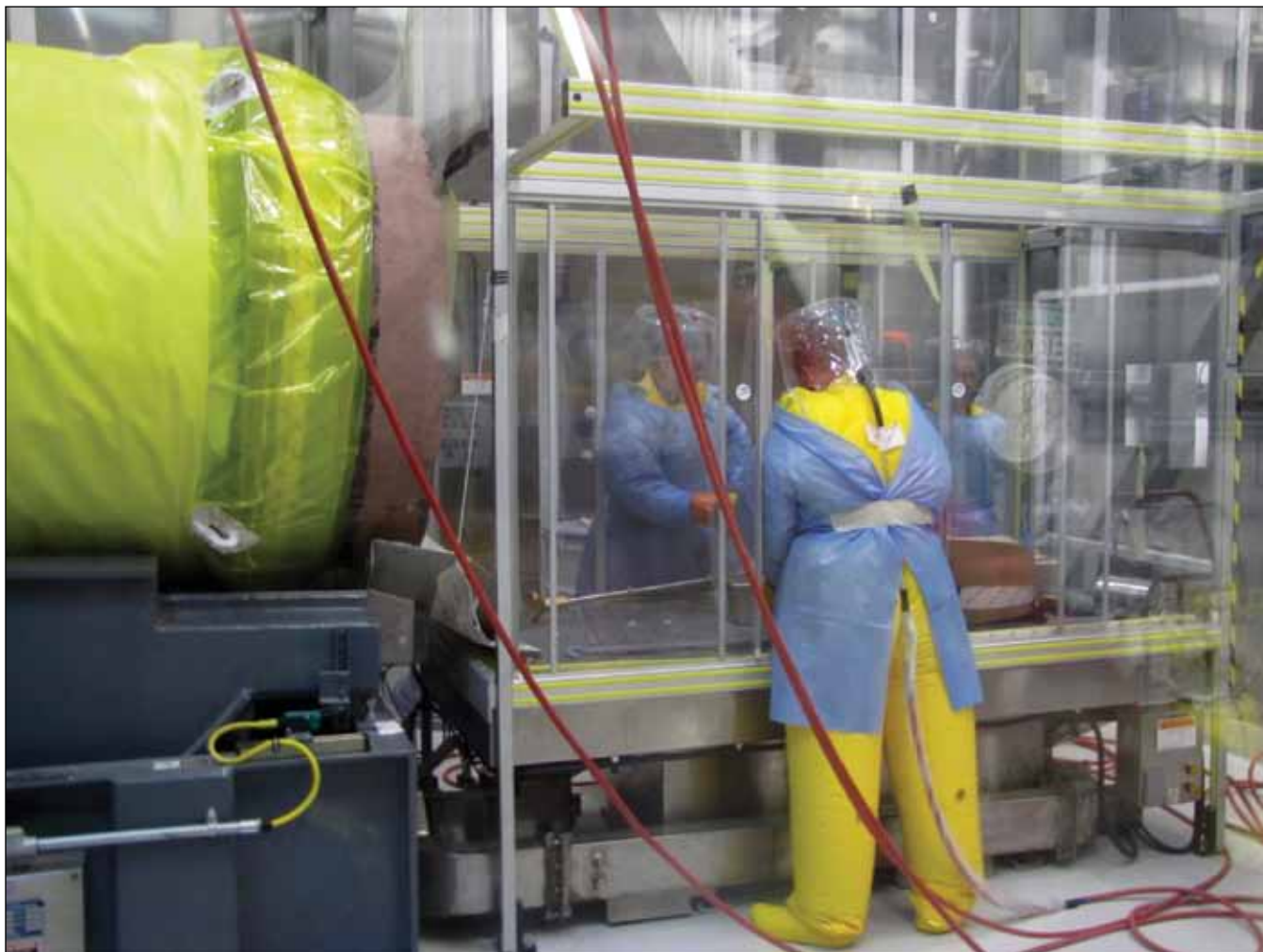
TWPC crew members work on cask waste on a table that allows for immediate groundwater separation from wastes.
