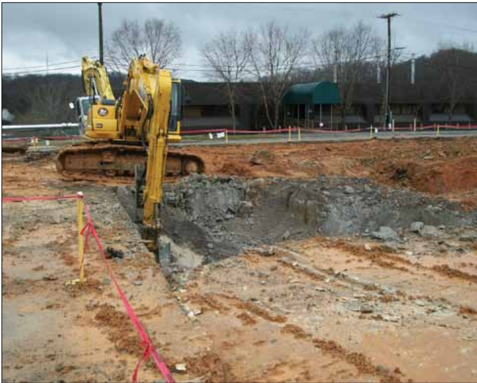
Pits beneath the Building 2000 slab are being remediated
