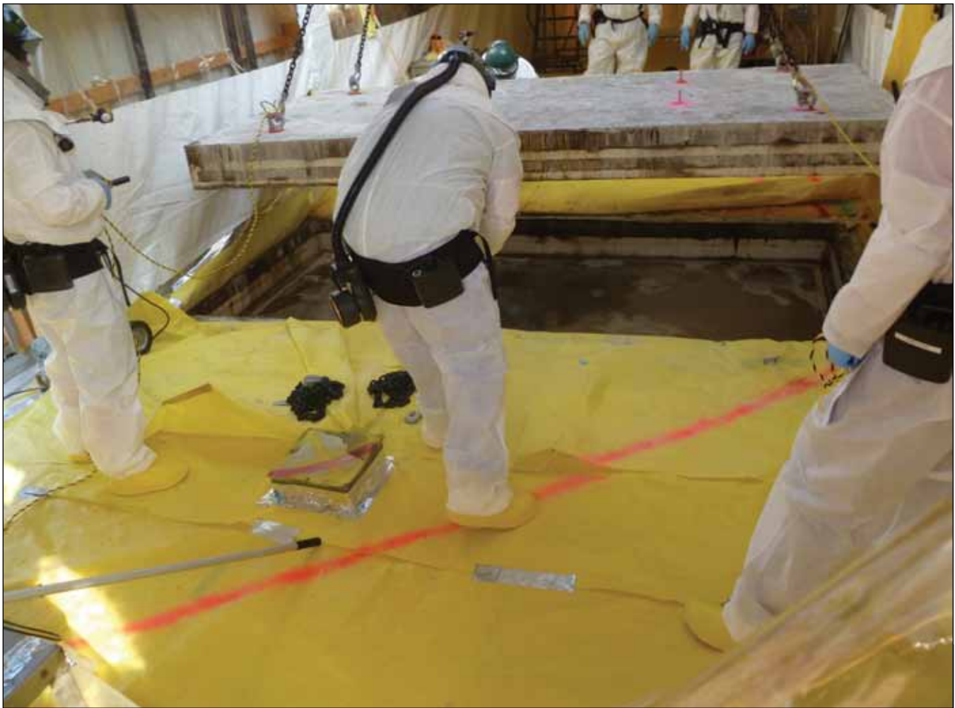
Workers are preparing to remove shield plug from a hot cell in Building 3026D
