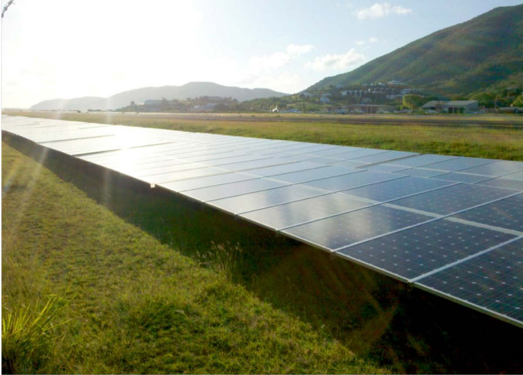
Figure 18. 451 kW PV system at Cyril E. King Airport on St. Thomas
