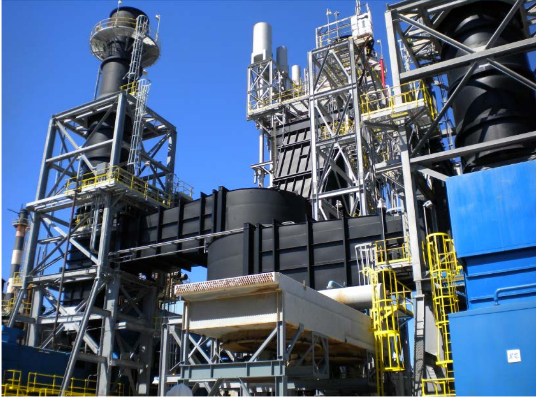
Figure 12. Heat recovery steam generators on St. Croix
