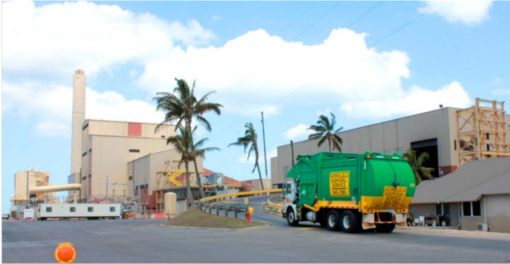
Figure 20. 50 MW waste-to-energy facility in Oahu, Hawaii
