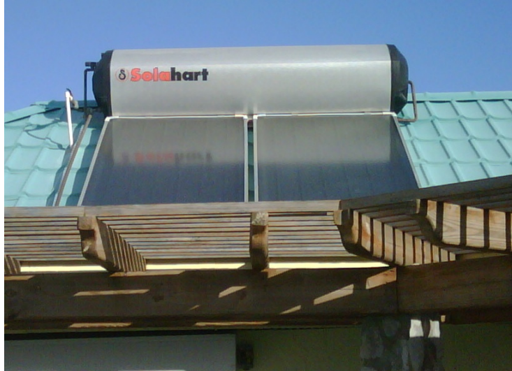
Figure A-14. Direct heat with integrated tank SWH system
