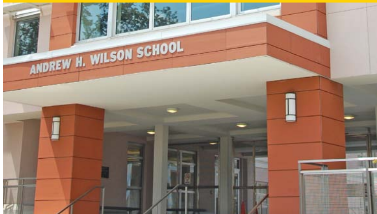
Andrew H. Wilson Elementary School, built in 1909, underwent a major renovation following Hurricane Katrina after suffering major flooding and wind damage. In addition to renovating the existing building, the school doubled its square footage and added both photovoltaic and solar hot water systems. Photo by Joe Ryan, NREL/PIX 19648
