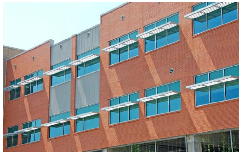
The majority of classrooms at Lake Area High School utilize daylighting thanks to the use of exterior shading and semi-transparent daylight glazing on the upper half of south-facing windows. Photo by Joe Ryan, NREL/PIX 19627
