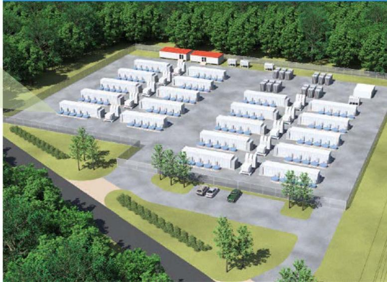
**Figure C-10. Concept of 20-MW frequency regulation plant**
