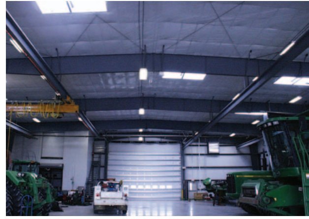
The insulated garage door and skylights at the BTI-Greensburg service center make this large, open area very energy efficient.
