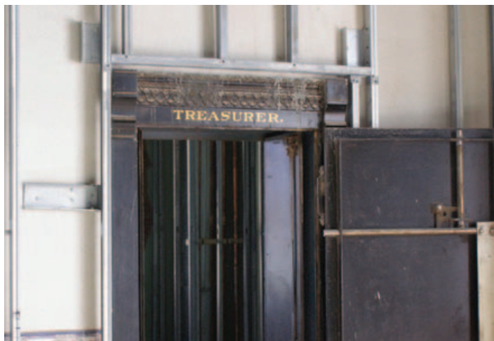
In rebuilding the Kiowa County, Kansas, courthouse—originally constructed in 1914—the community decided to salvage the original white trim along with several ornate doors from the stately and historic building.
