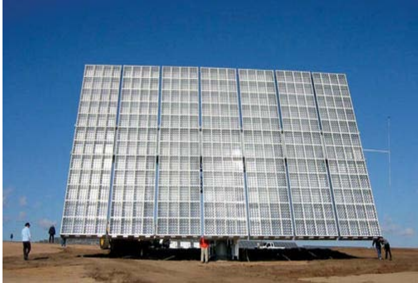
Figure 4. Typical utility-scale concentrating PV system (NREL PIX 13735)
