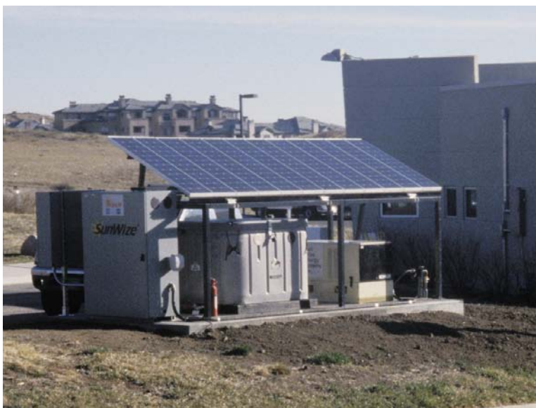
Figure 10. A PV UPS system at NREL that supplies electricity to XCEL Energy during normal operation and emergency power to the laboratory during power interruptions (J. Thornton).
