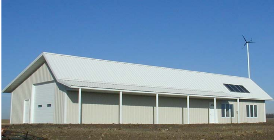
Figure 11. A wind farm maintenance shop in Woodstock, Minnesota that uses a hybrid wind and PV system as a source of power
