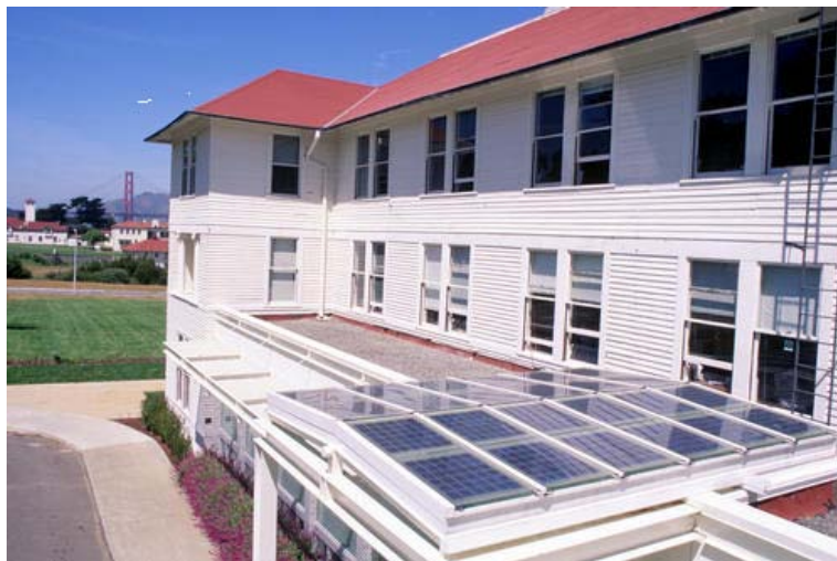
Figure 6. PV modules being used as an overhead shade on a commercial building
