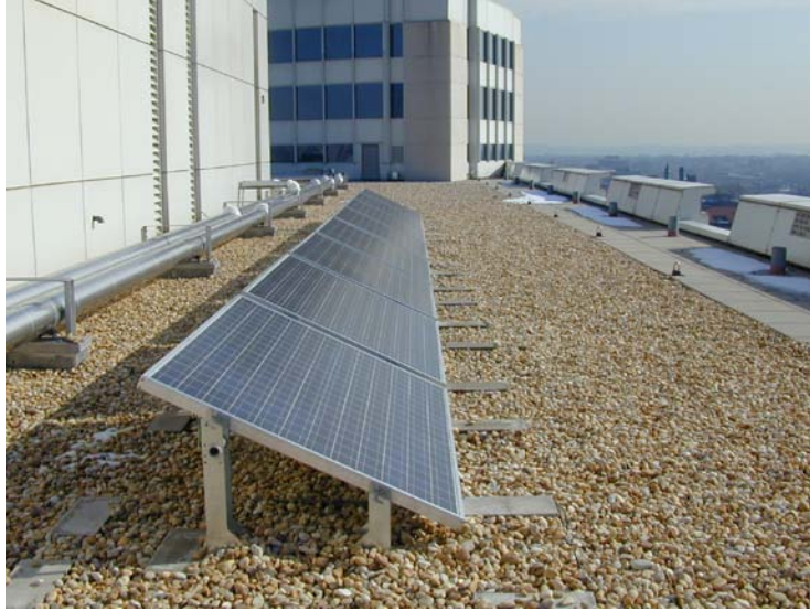
Figure 2. Typical fixed-tilt, non-tracking, flat-plate PV system (J. Thornton)
