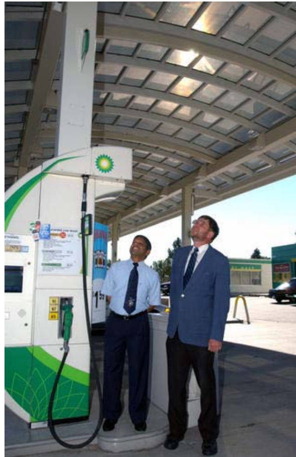
Figure 7. PV canopies are often used to shade gasoline pumps at service stations. (NREL PIX 11979)
