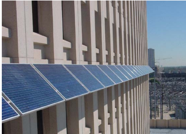
Figure 5. PV modules being used as awnings to provide shade as well as electric power
