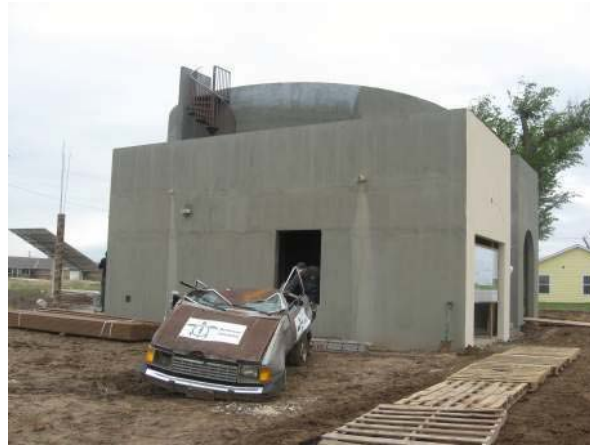
Figure 25. The Silo Eco-Home is built similarly to a grain silo, which was one of the few structures left standing in Greensburg after the tornado. On April 9, 2009, the builder (Armour Homes of Bushnell, Florida) tested the home's ability to withstand pressure by dropping a 1980 Honda Civic on the roof from a height of 60 ft. The home, unlike the car, was undamaged.
